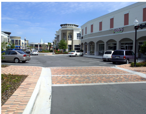
Decorative pavement used at crosswalks to slow traffic and cue motorists of crossing pedestrians
