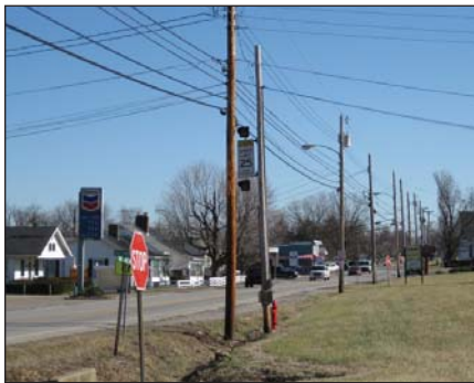
Overhead utilities, drainage, no sidewalk
