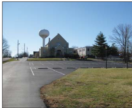
Large parking area fronts US 60
