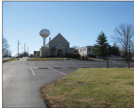
Large parking area fronts US 60
