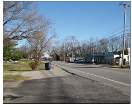
No sidewalk, unrestricted access
