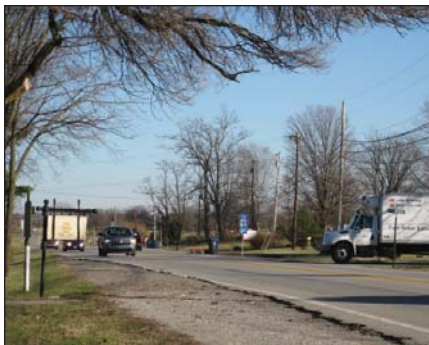
US 60 corridor (looking east)
