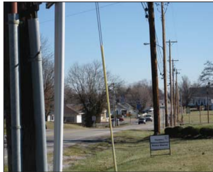
No sidewalk, overhead utilities
