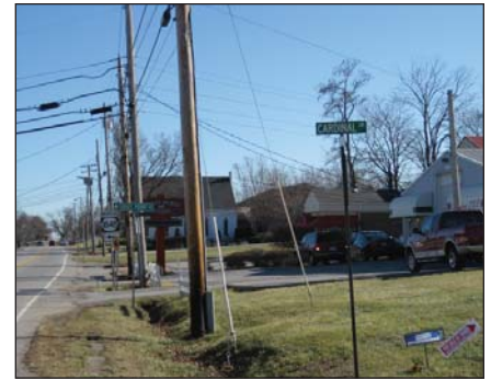
Multiple access points, overhead utilities, drainage, pedestrian desire line observed
