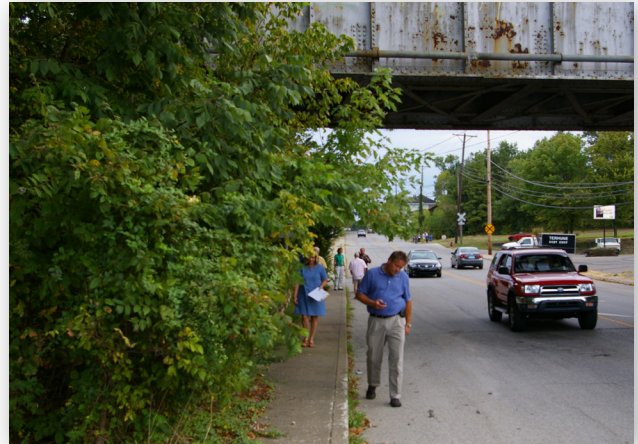
Poor maintenance of existing sidewalks, such as failure to remove obstructions, contributes to poor mobility
