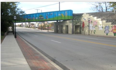
Preston Highway Railroad Bridge, Louisville, Kentucky, after renovation
