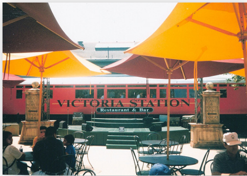
Rail car adaptive reuse examples. Victoria Station is an international chain of rail car themed upscale restaurants.
