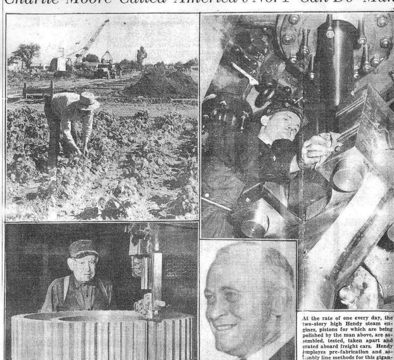
They wasted no time converting a string bean field into a pulsating machine building at Joshua Hendy Iron Works in Sunnyvale. Upper picture shows a bean picker hurrying his job while workmen follow up laying foundations for the buildings. Lower photo shows a gear being finished up in the building for one of Hendy's 274,000-pound triple expansion engines—the heartbeats for Henry Kaiser's Liberty fleet.
