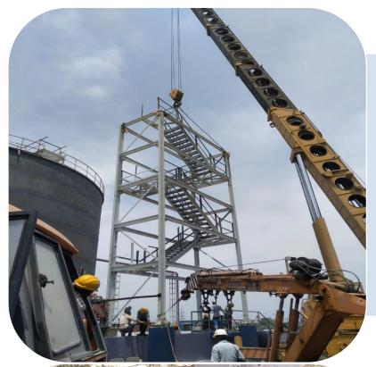
Staircase assembly and erection with single lift
