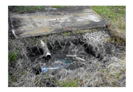
An exposed septic tank pit filled to ground level with nasty looking backed-up septic tank waste.
