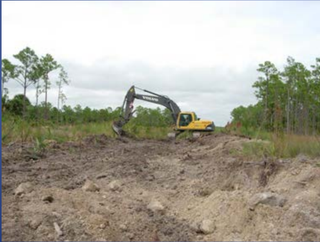
Removing berm and backfilling agricultural ditch
