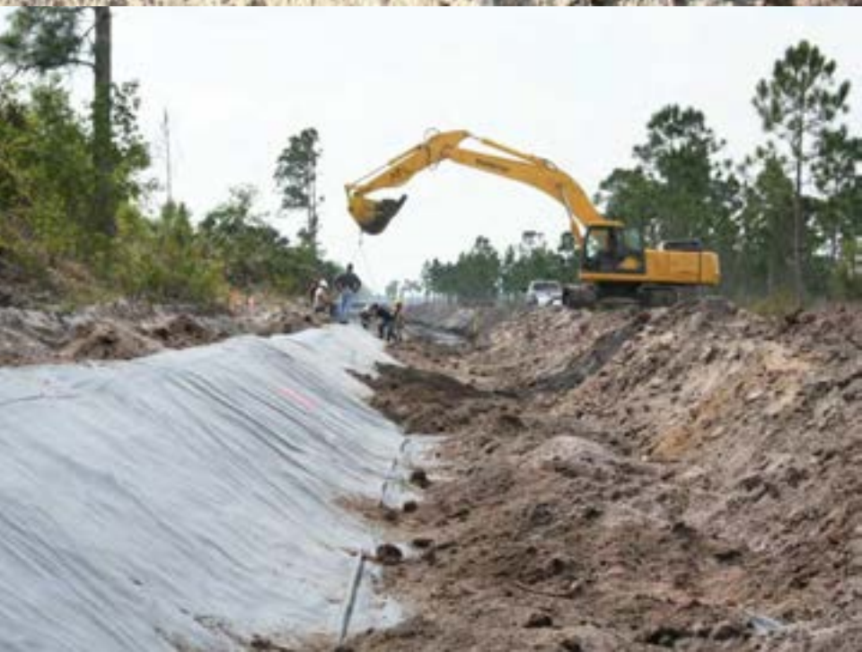
Seepage Barrier Installation – Spring 2011
