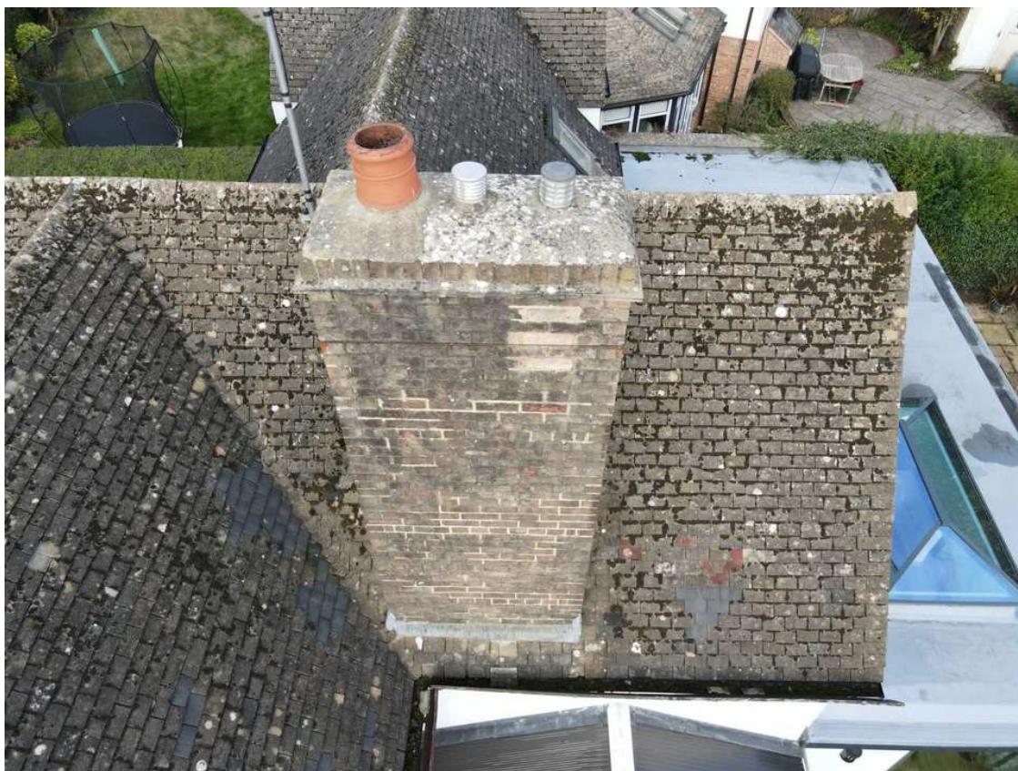
General view chimney stack.
