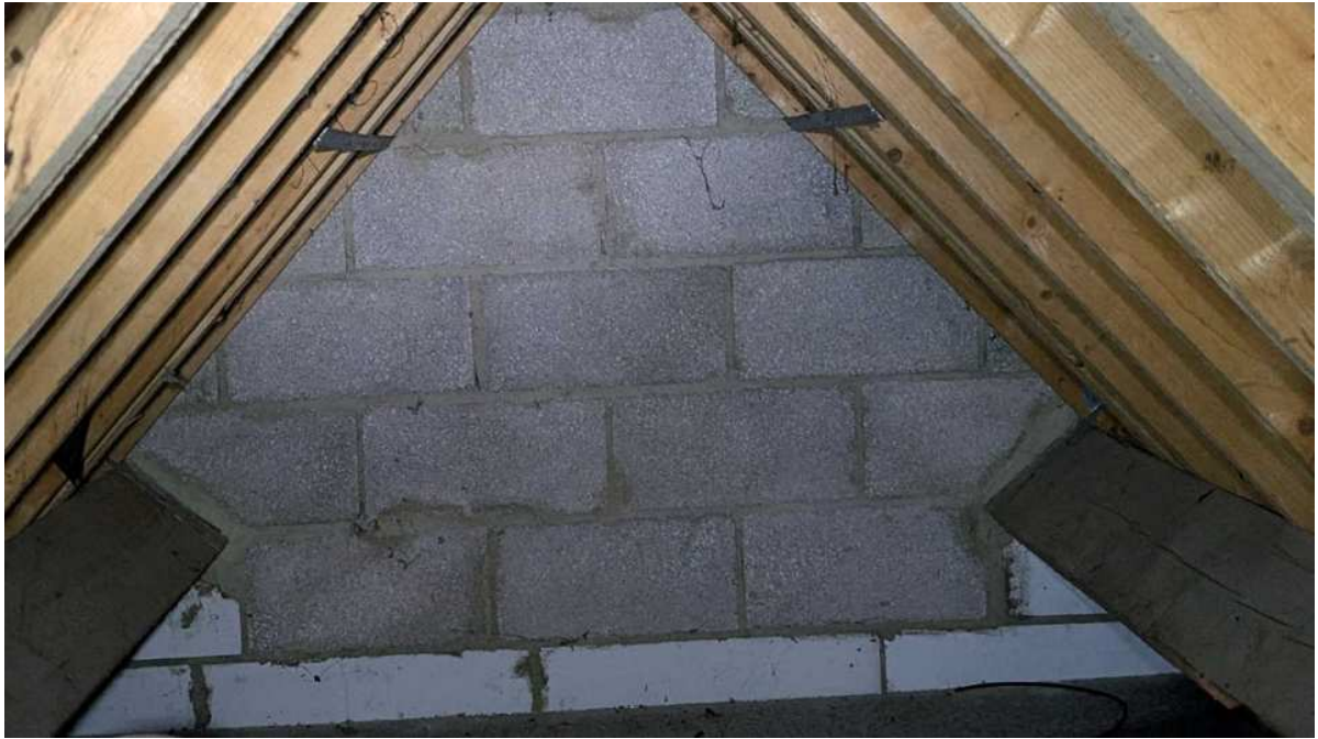
Blockwork free from cracking.
