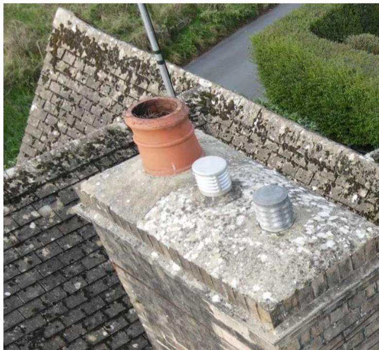
Flue servicing living room and capped flues.
