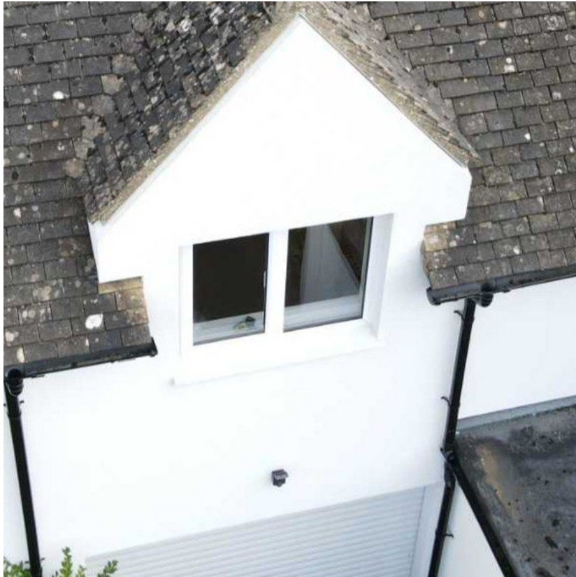
PVCu guttering across the roof.
