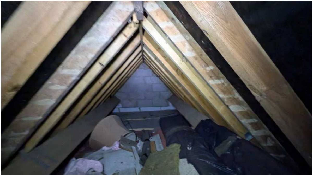
Roof space facing the extension.
