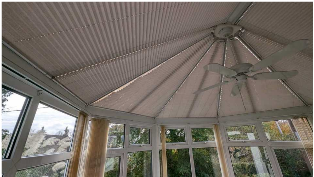
Framing and blinds: general view.
