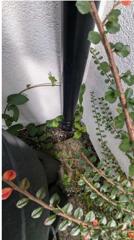
Downpipe adjacent to Hall.
