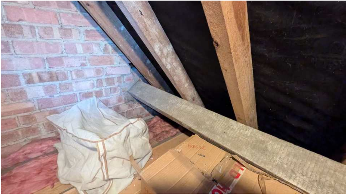
Existing rafter and purlin formation.
