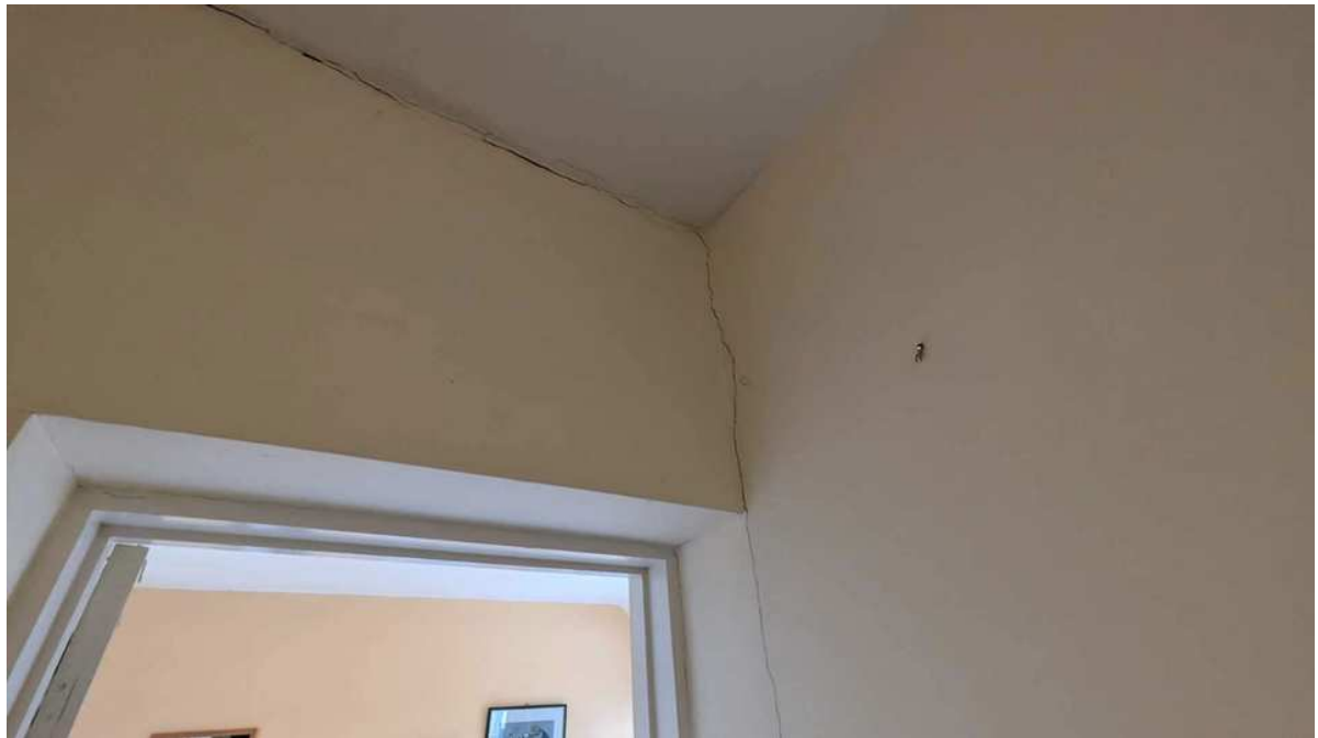
Cracking between original build and extension.
