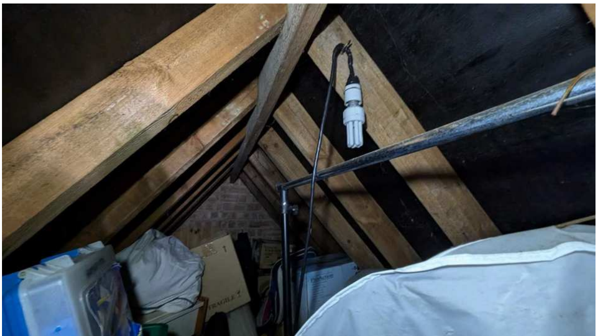
Roof space over bedroom 2.
