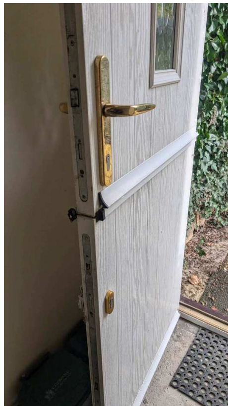
Stable door from garage to garden.
