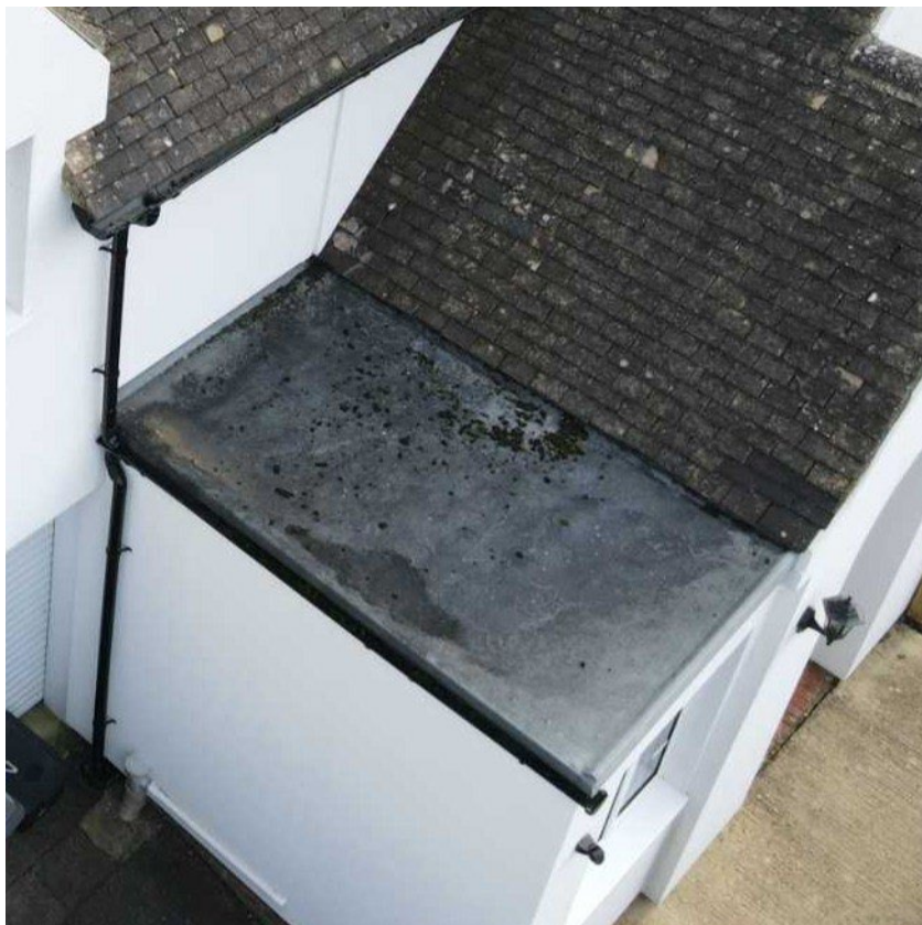
Ground floor toilet roof.
