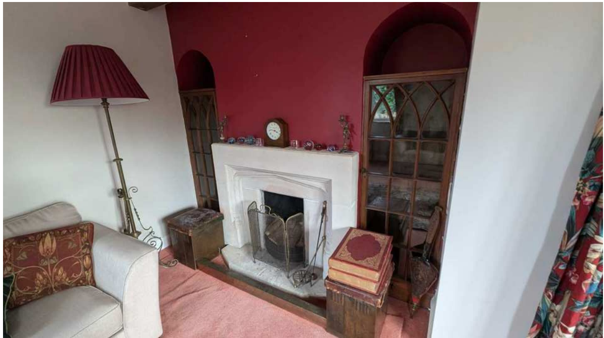
Potential for damp at the base of the fireplace.
