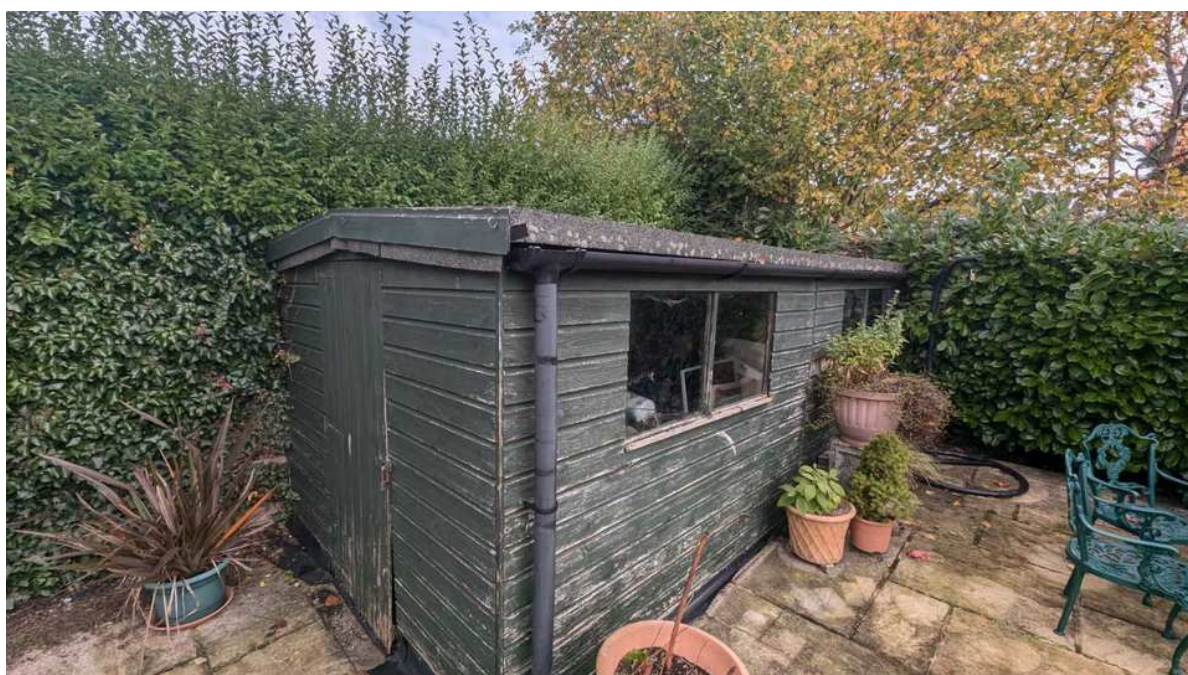
General view shed.
