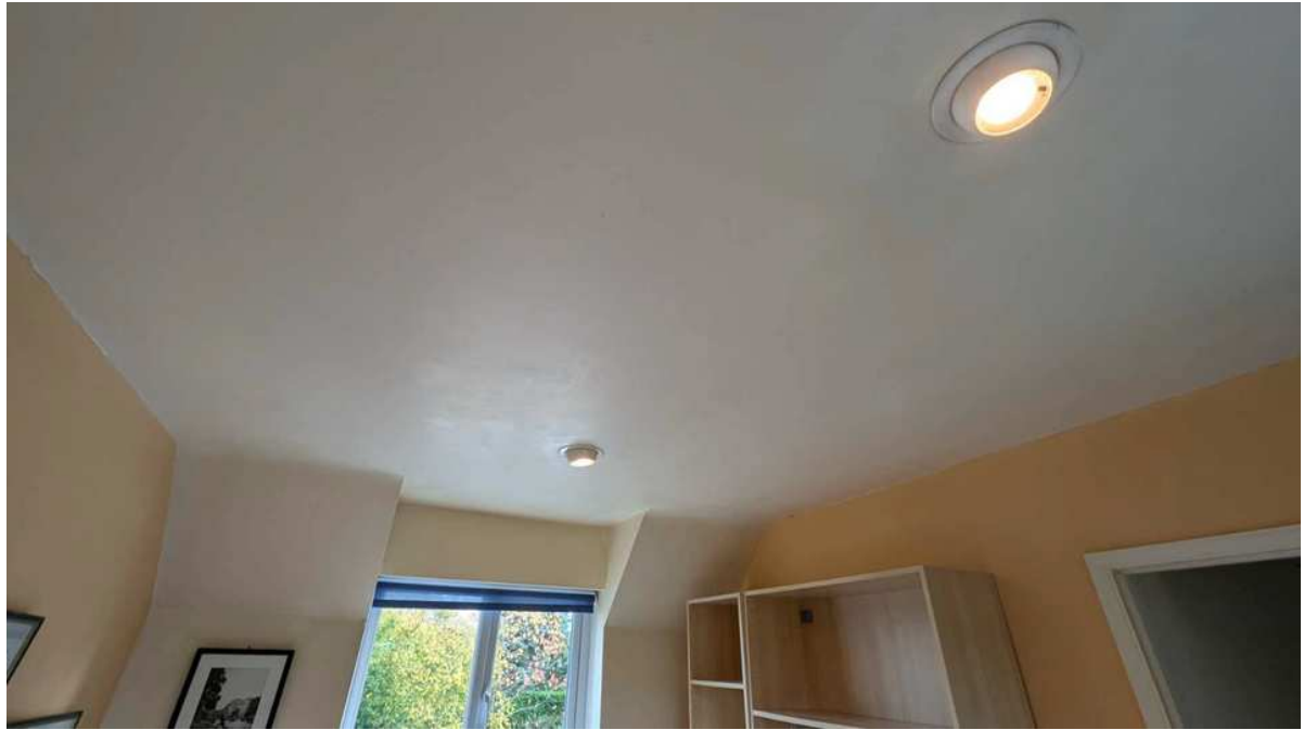
Gypsum plastered ceiling free from cracking.
