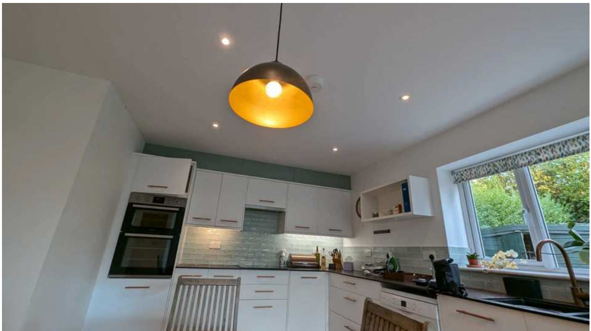
Gypsum plastered ceiling free from cracking.
