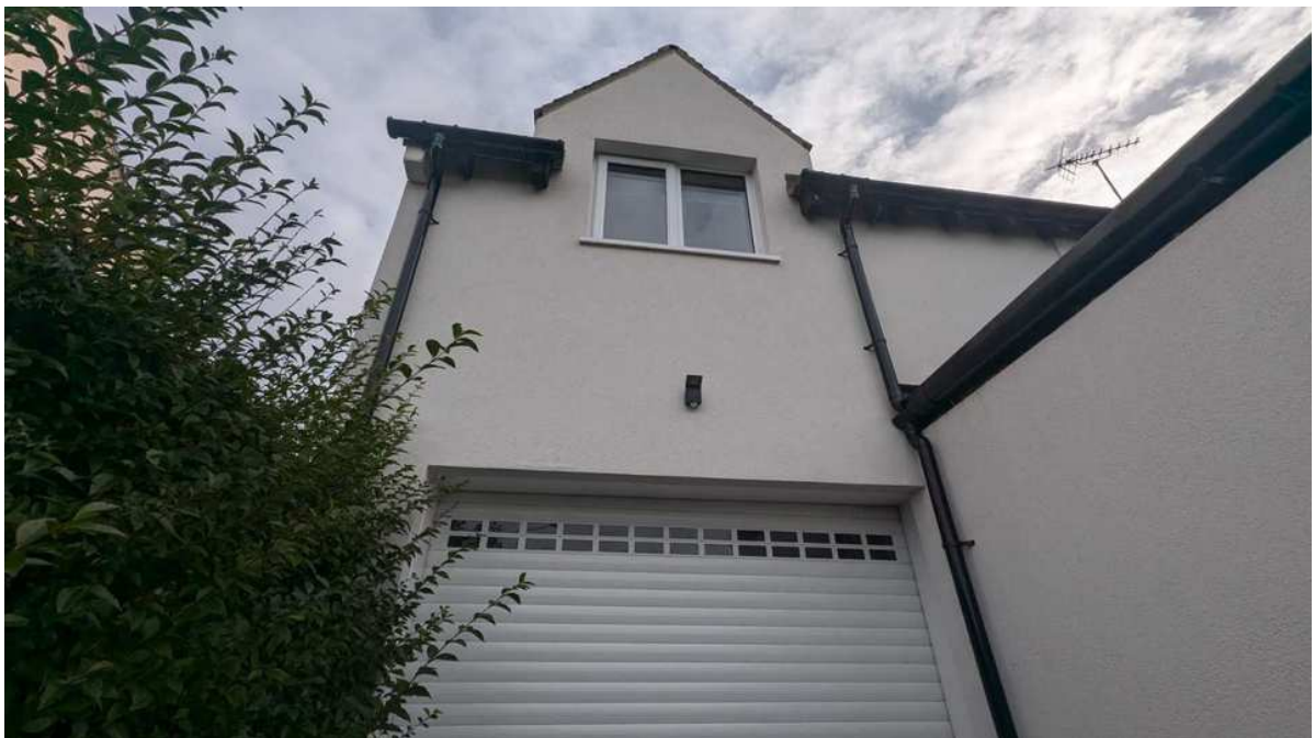
View of front elevation extension.
