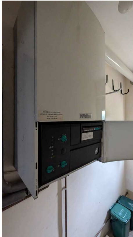
The boiler appears to be an old installation.
