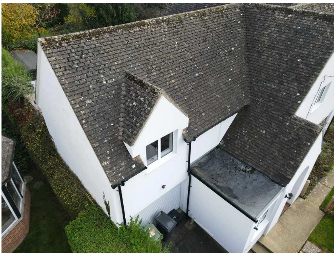
The left hand gable view of the roof.
