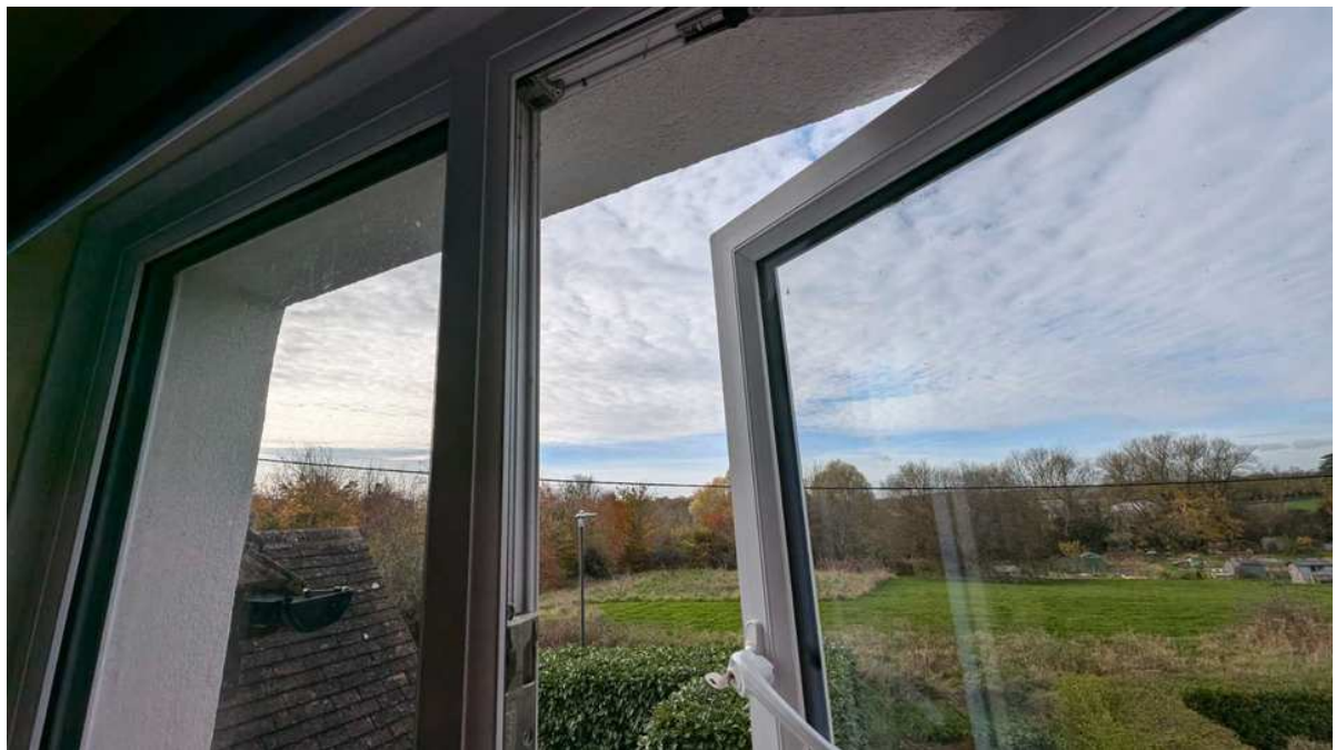
Upper floor windows.
