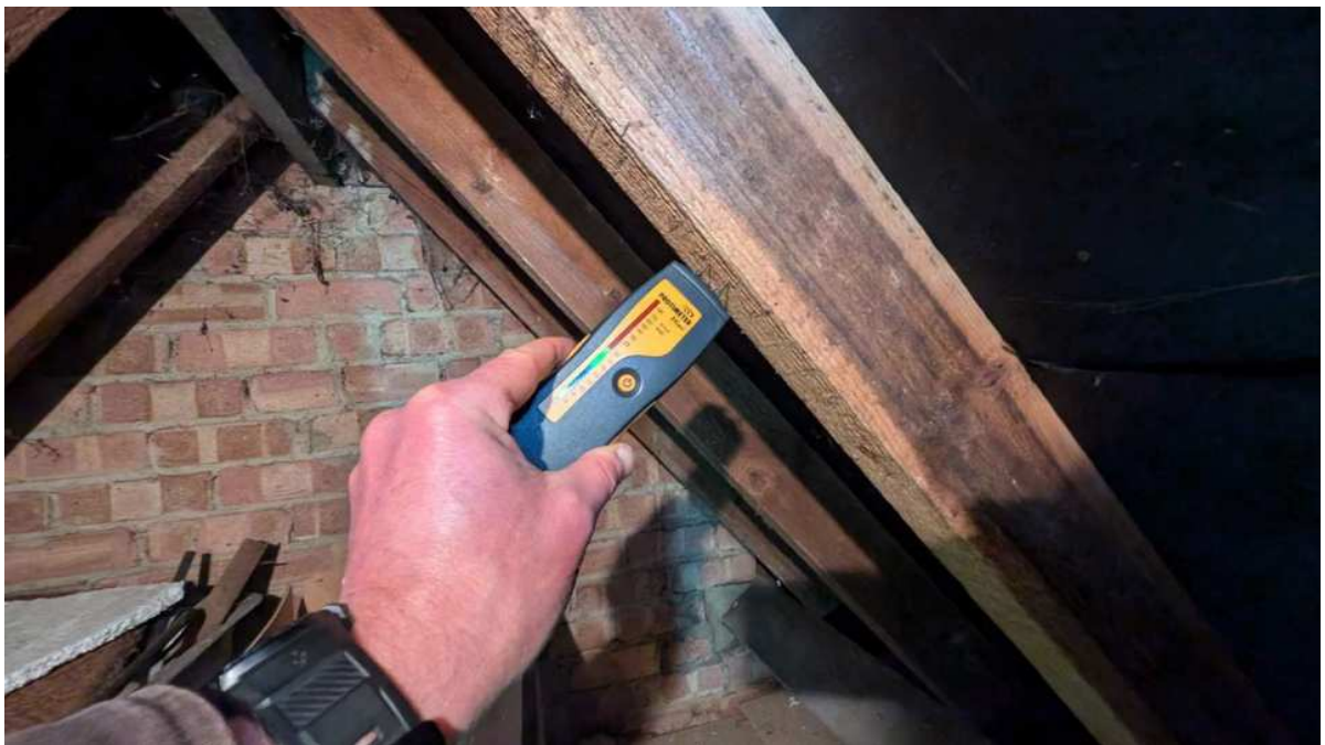
Roofing Timbers : acceptable moisture level.
