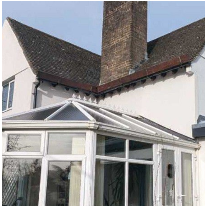
Exposed rafter shoes and snow guard.
