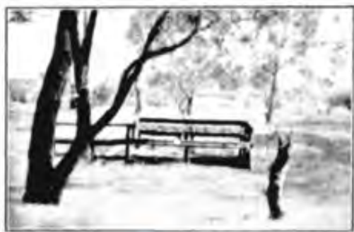
Northam's first water supply came from this well, located at the Aboriginal Reserve. Source — Western Mail, September 21st, 1933
