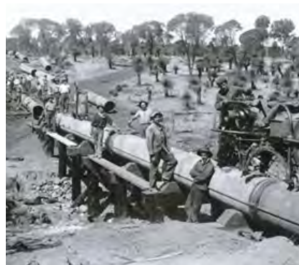
Construction of the pipeline for the Goldfields Water Supply Scheme. Source — State Library of WA
