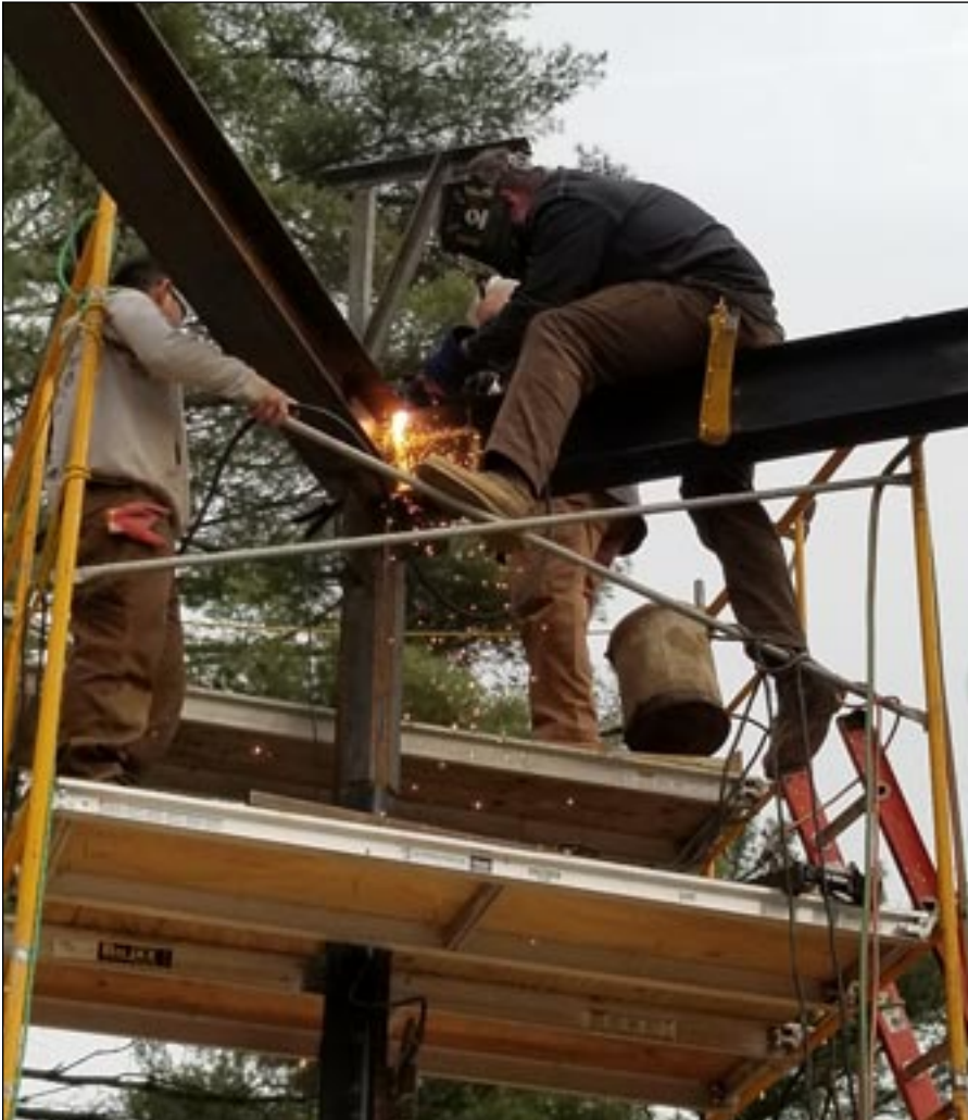
Phoenix, MD In Progress — Photo: Centurian Construction
