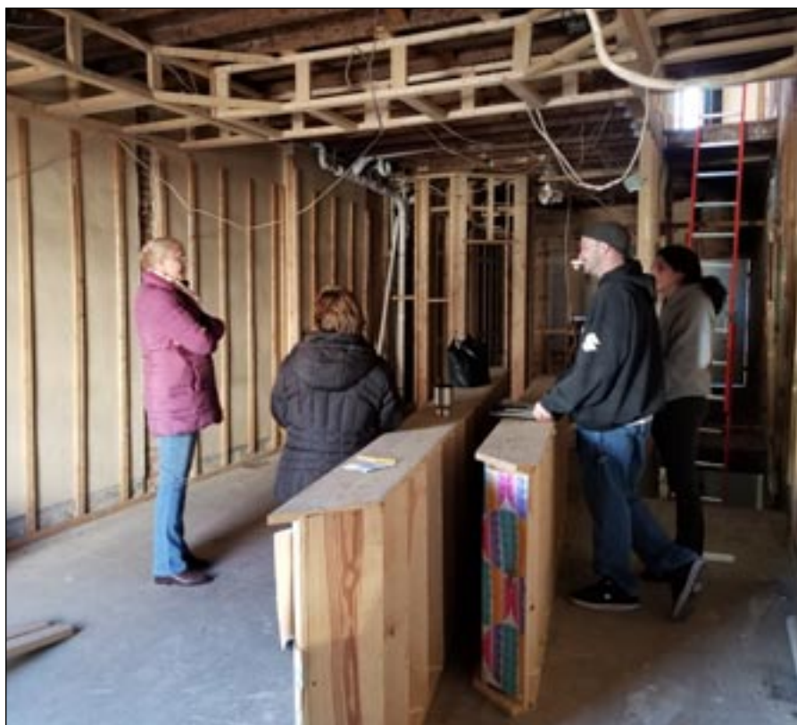
N. Luzerne Framing In Progress — Photo: Centurian Construction
