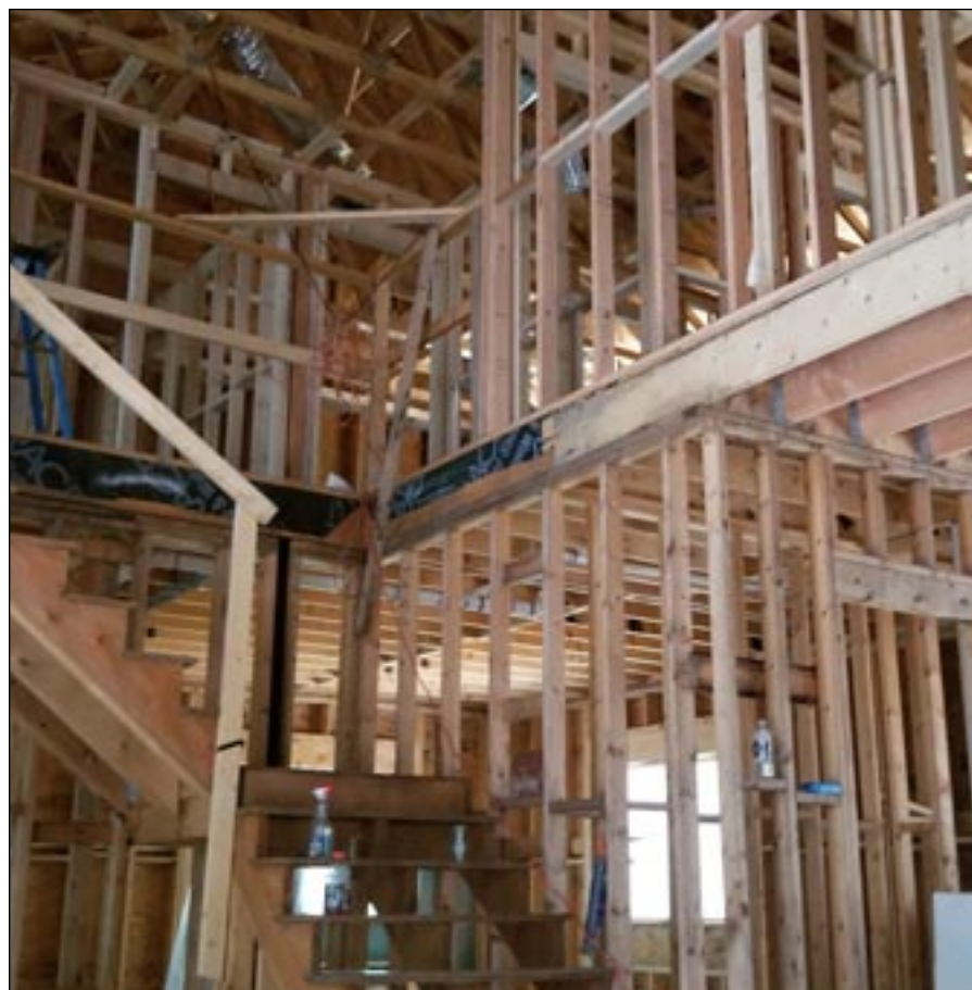
Manor Road In Progress — Photo: Centurian Construction
