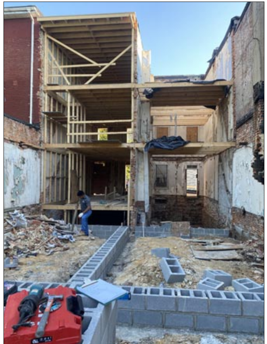
McHenry Street In Progress — Photo: Centurian Construction
