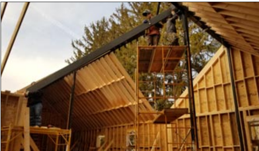
Phoenix, MD In Progress — Photo: Centurian Construction
