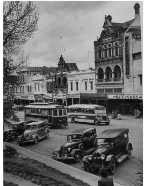
Note the tram "Special" and the bus design with the driver seated behind the engine
