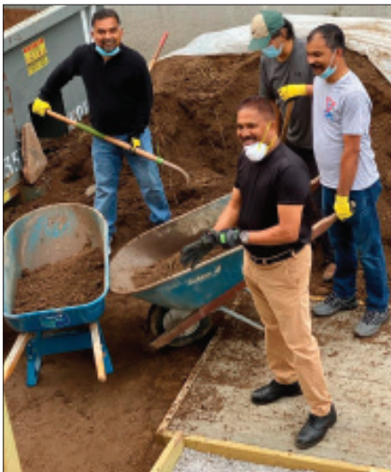
Joining hands with Habitat for Humanity in building a house for the less privileged
