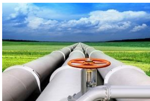
Hydrogen Pipeline; Image: UNECE
