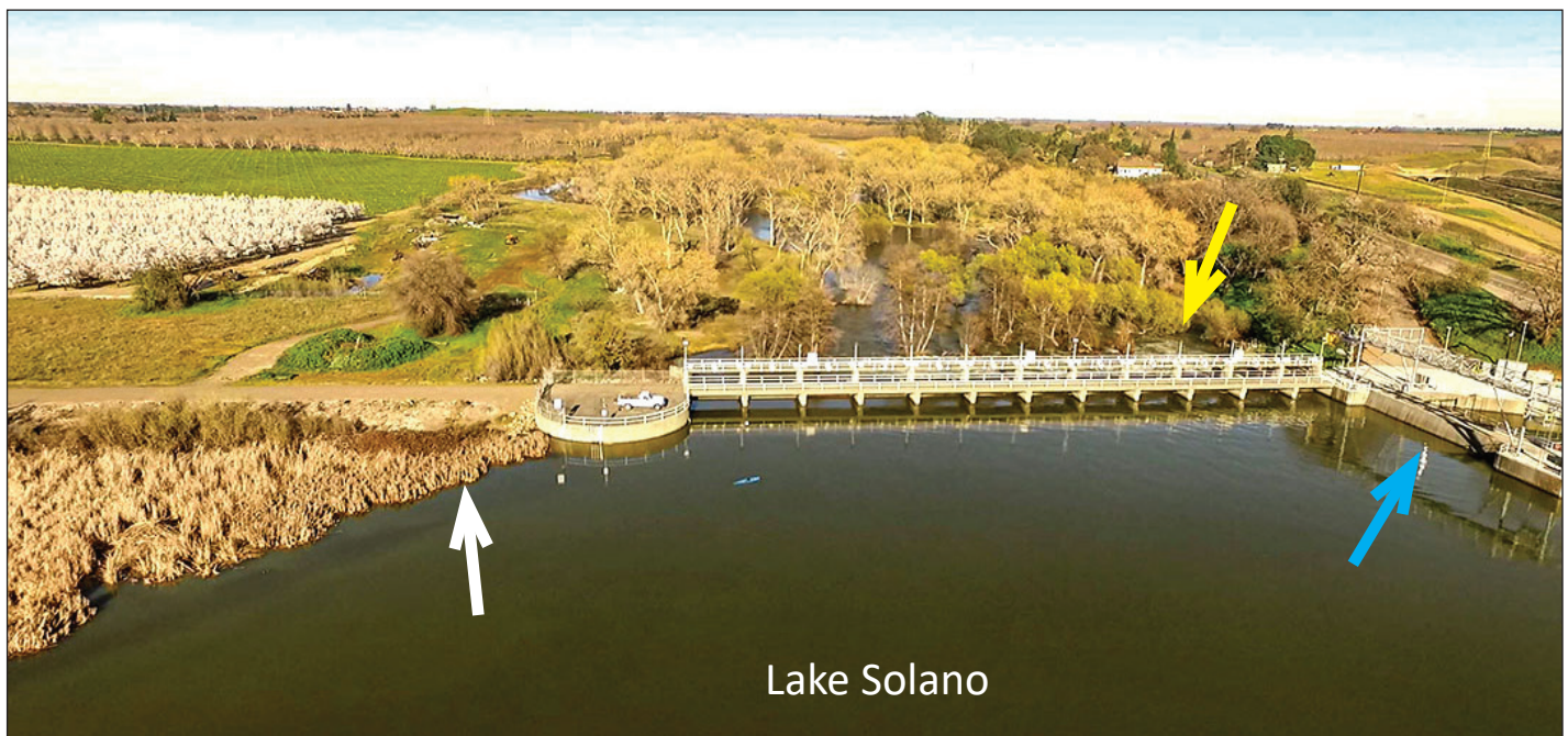
Putah Diversion Dam and Lake Solano on 3/24/2017. Image from aerial video during high-water event shows the Diversion Dam and Lower Putah Creek. Arrows show the soft plug (white arrow), Lower Putah Creek (yellow arrow) and the entrance into the Putah South Canal (blue arrow).
