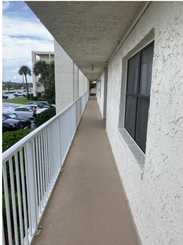
Photograph #8 – Typical walkway corridor
