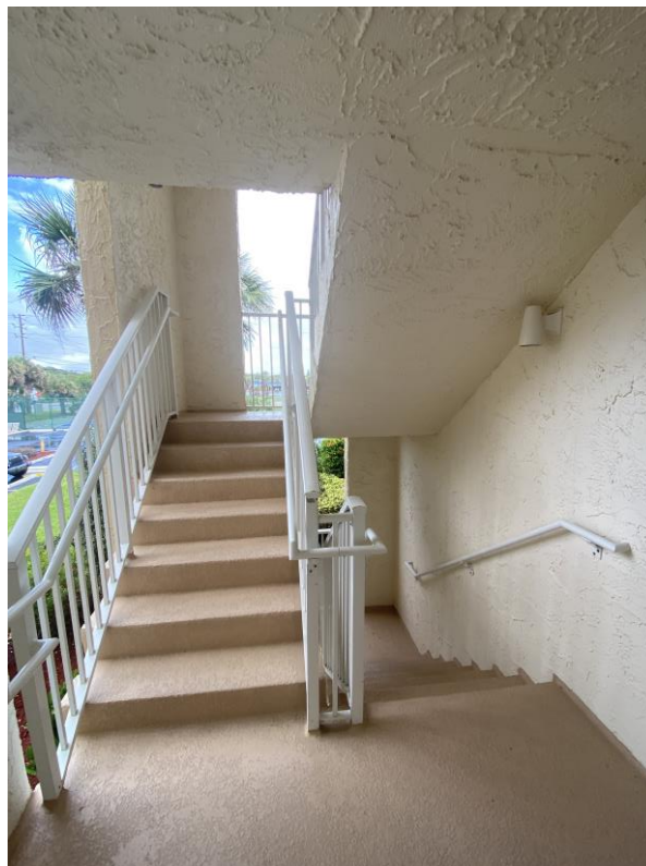
Photograph #9 – Typical stairwell
