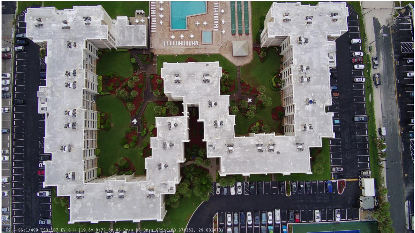
Photograph #5 – Roof layout aerial photograph
