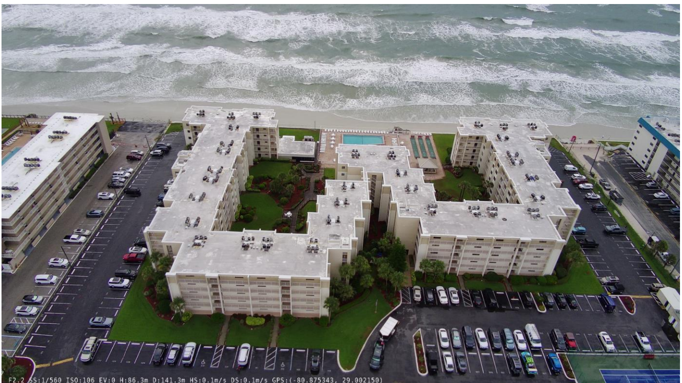
Photograph #2 – West elevation aerial photograph
