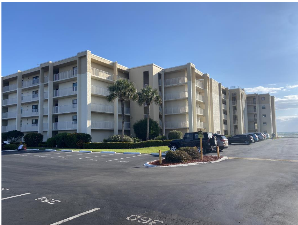
Photograph #5 – Typical walkway elevation (Southwest)
