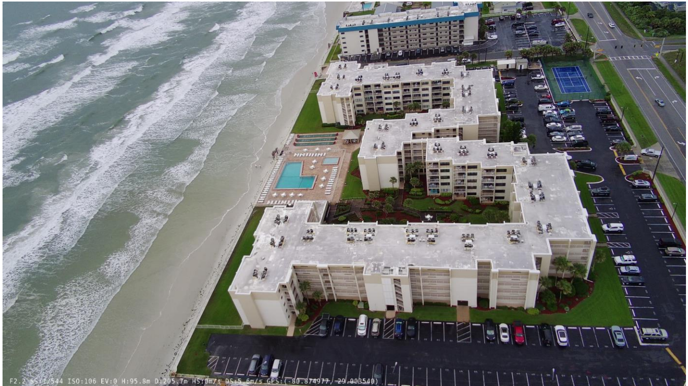
Photograph #3 - North elevation aerial photograph
