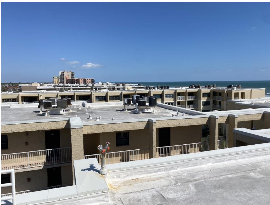
Photograph #11 – Typical roof layout
