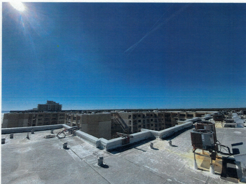
Picture 8: Typical roof
