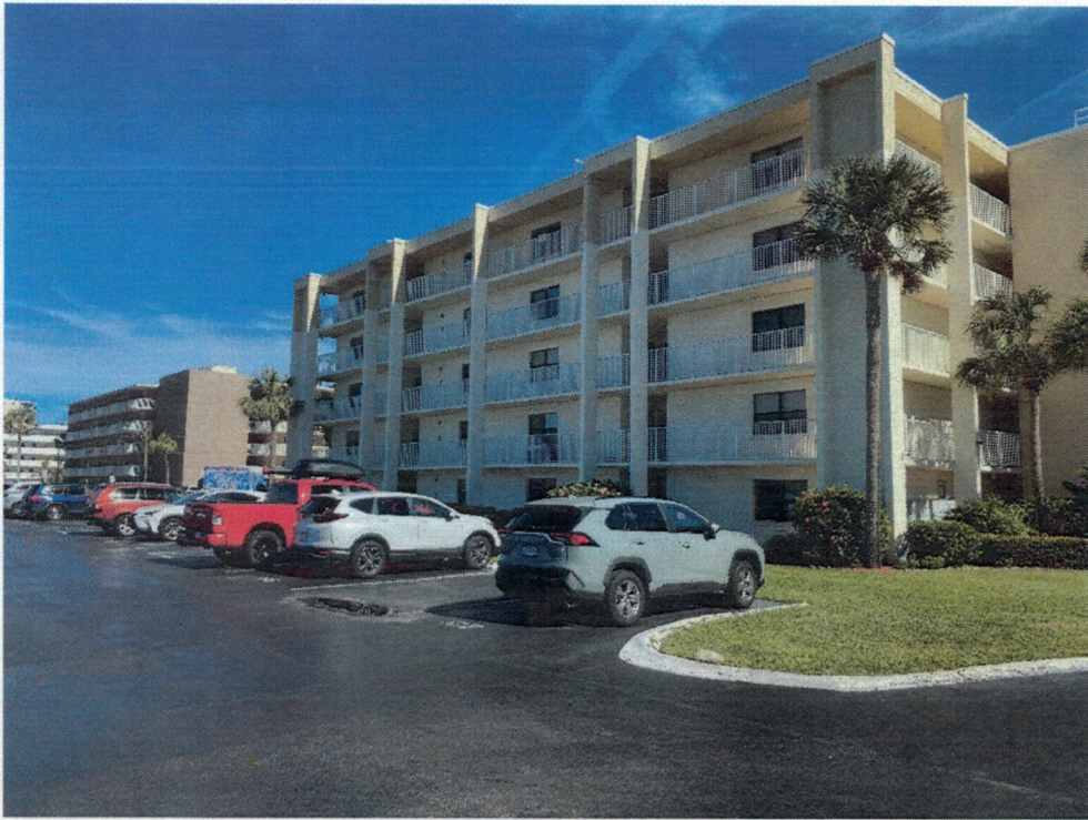
Picture 5: West elevation of building
