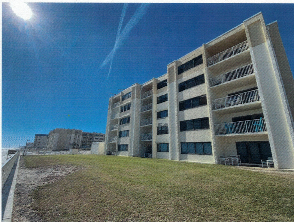
Picture 3: East elevation of building
