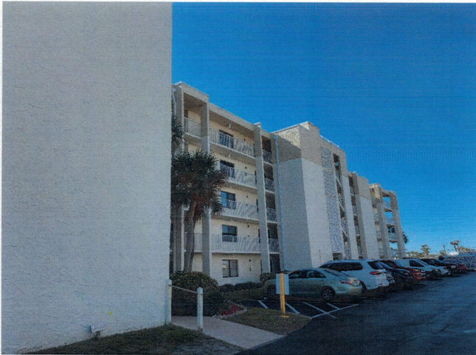
Picture 2: North elevation of building
