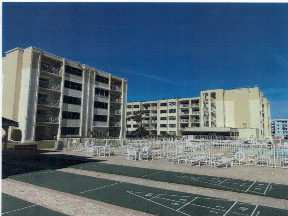
Picture 4: East elevation of building
