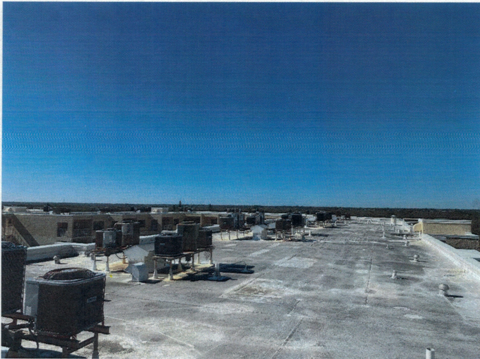
Picture 6: Typical roof
