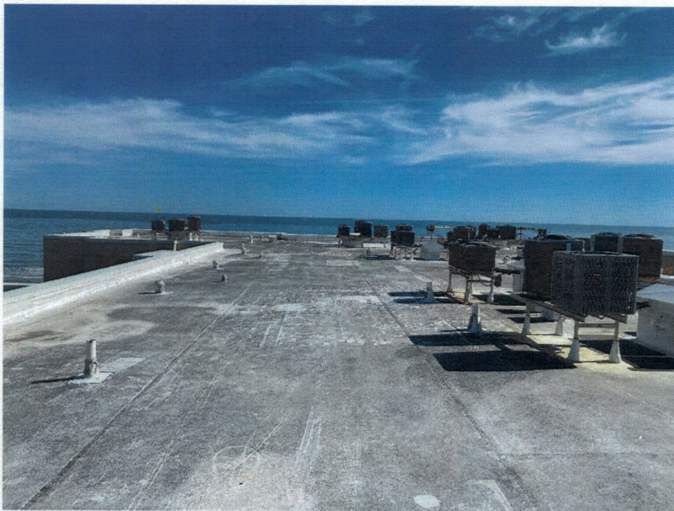
Picture 7: Typical roof
