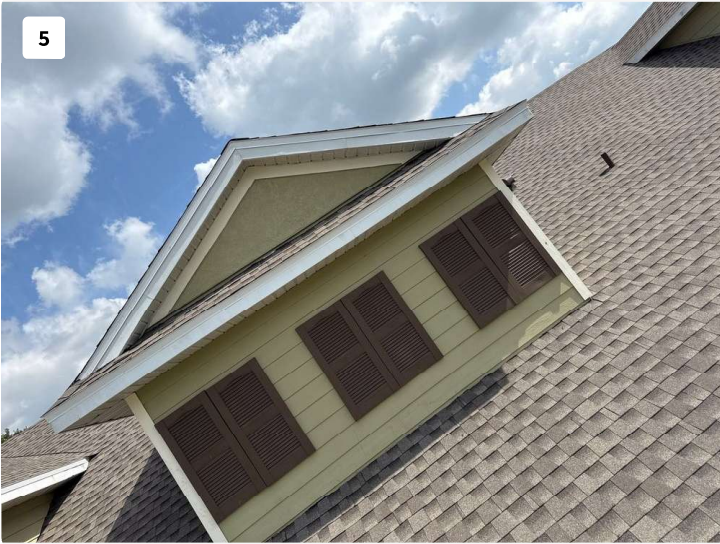
Project: Hammocks 2- Broken Willow 8508-8514 / 2412-6437700-01 Date: May 1, 2025, 10:32 AM Creator: Jose Luna
