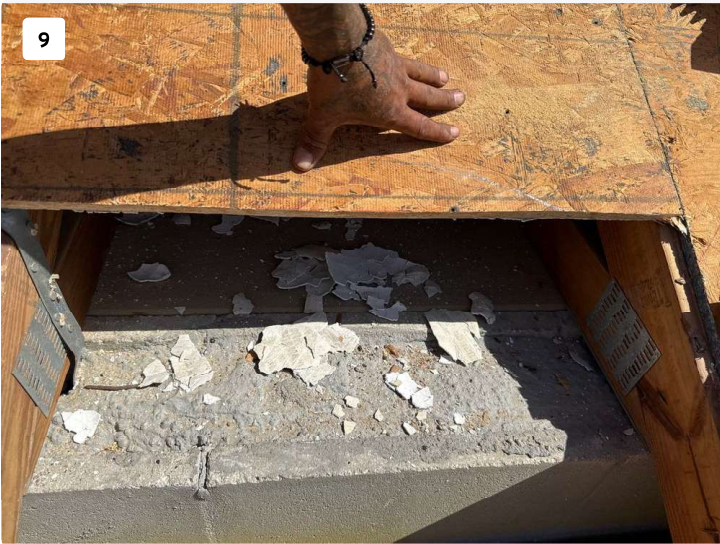
Project: Hammocks 2- Broken Willow 8508-8514 / 2412-6437700-01 Date: Apr 30, 2025, 11:07 AM Creator: Jose Luna
