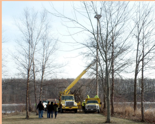
REMC crew place pole and platform in ground.
