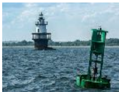
Hog Island Shoal Light Hog Island, RI (1901-current) Example of caisson style lighthouse (Replaced 1886 Lightship)
