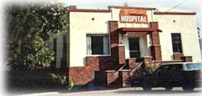
First Professional Hospital Building
