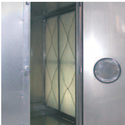
drop separator for high-pressure humidifier
