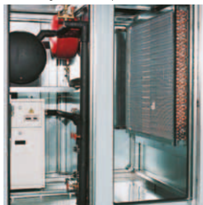
indirect cooling with cold water set
