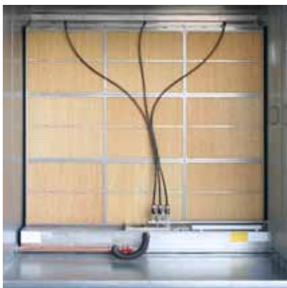
Contact humidifier with three cascades
