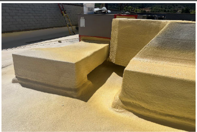
Seams and penetrations are the primary sources of leaks in a roof systems, spray foam eliminates this vulnerability
