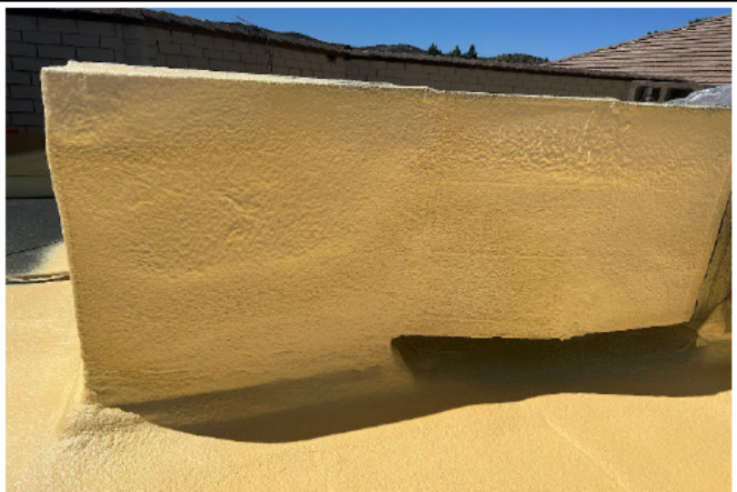
The surface is prep and sprayed with polyurethane foam
