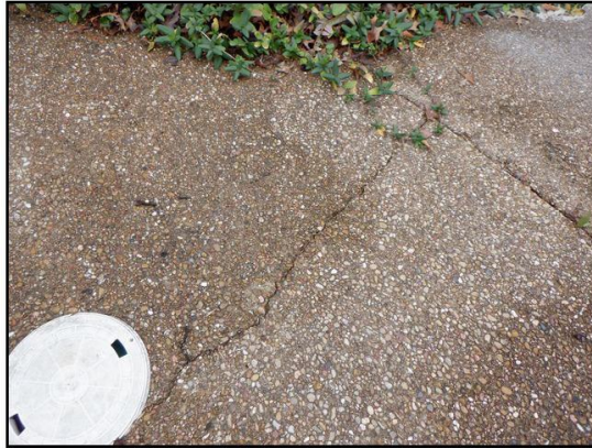
Typical cracks at exterior pool decking in various locations.
