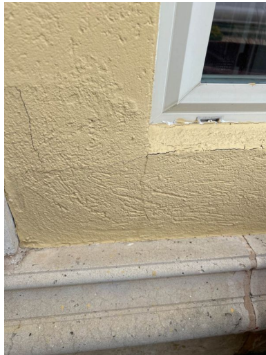
Cracks and Damage - Front Exterior
