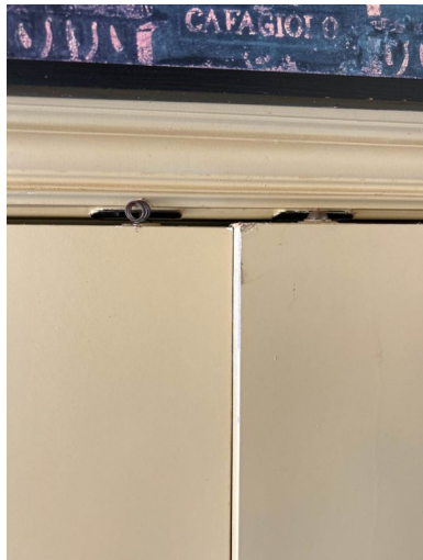
Garage Water Heater Closet
