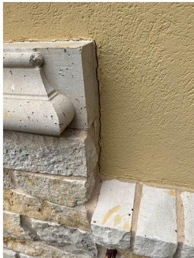
Cracks and Damage - Front Exterior
