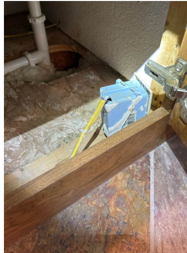
Master Bathroom under tub
