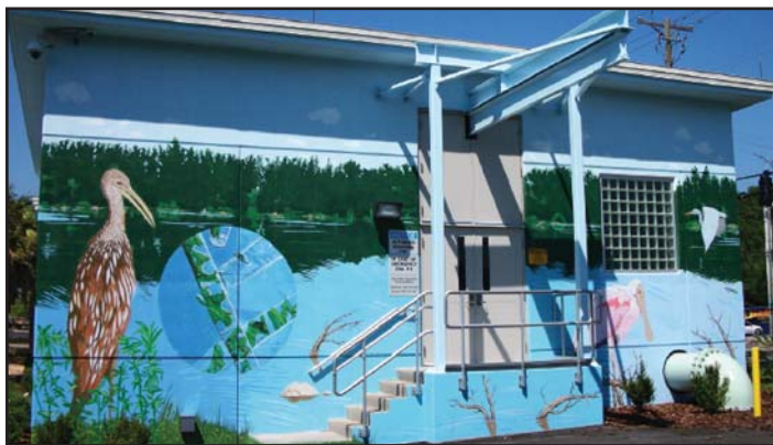
Figure 6. Sulphur Springs Pump Station building aesthetics were an important consideration because the facility is located within a municipal park.
