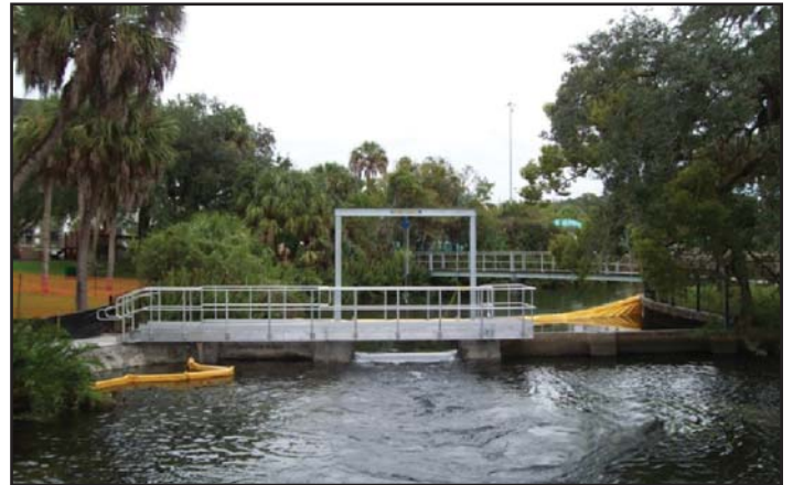
Figure 11. Rehabilitated Sulphur Springs Run Lower Weir (2011).
