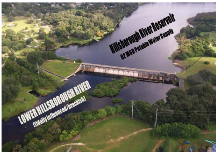
Figure 1. The Hillsborough River Dam impounds freshwater for the City of Tampa's water supply.
