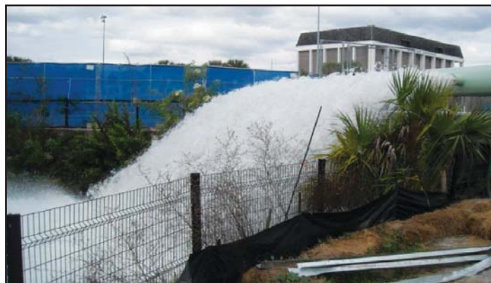
Figure 7. The new Sulphur Springs Run discharge header provides sufficient aeration to support downstream fauna.
