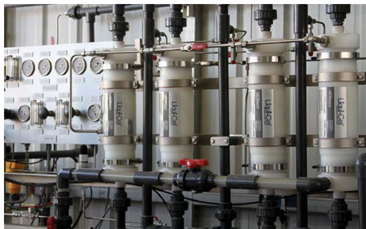
Membrane contactors remove dissolved oxygen to prevent arsenic mobilization.
