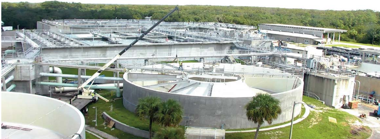
New 316 stainless steel effluent launders installed in Unit 1, Process Train 2 increasing hydraulic capacity of the Train 2 solids contact unit (SCU) from 6 mgd to up to 8 mgd. Note the pentagon structure on the left side. (photo: Kevin Morris, PRMRWSA)
