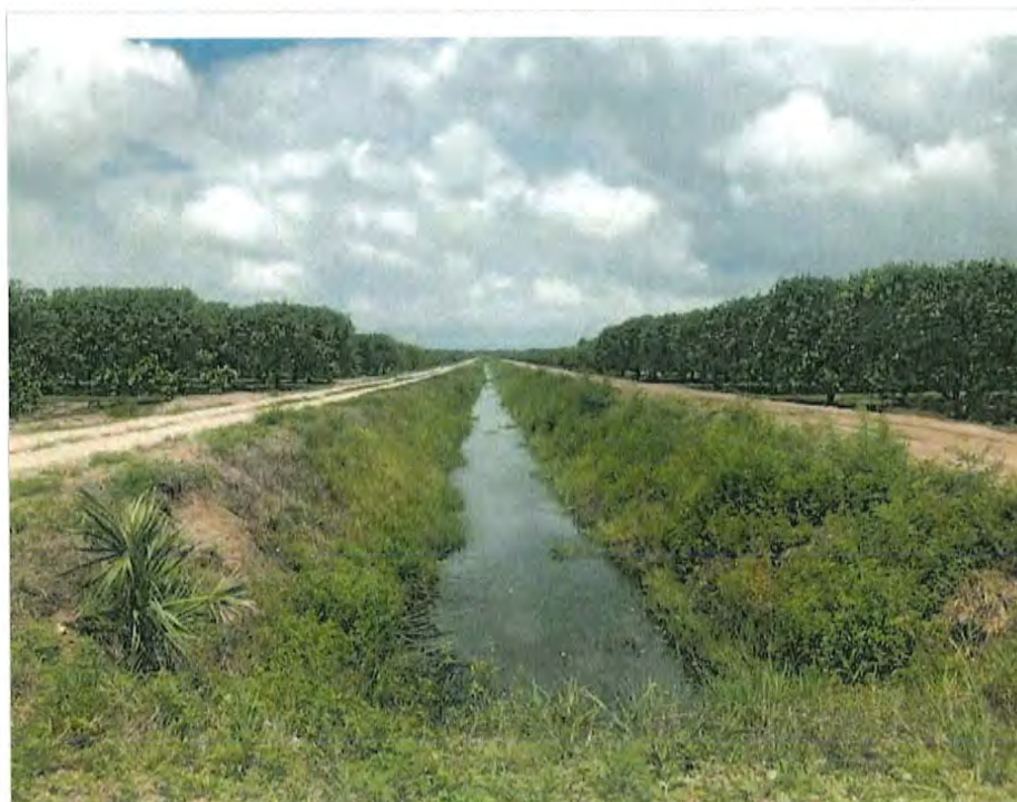
SUBJECT'S DRAINAGE SYSTEM
