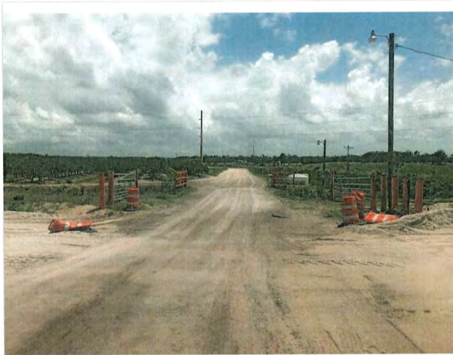
SOUTHERLY VIEW OF SUBJECT'S DRIVEWAY CONNECTION ALONG SR 82
