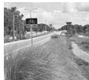
Bioswales are planted swales that provide treatment and retention of storm-water. (EPA Green Infrastructure ).
