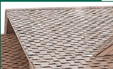
Figure 5-2: Reinforced asphalt shingles
