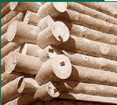
Figure 5-7: Log wall construction
