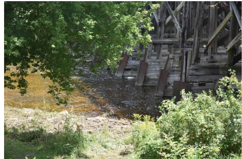
Debris at the base of bridge footings were also removed.
