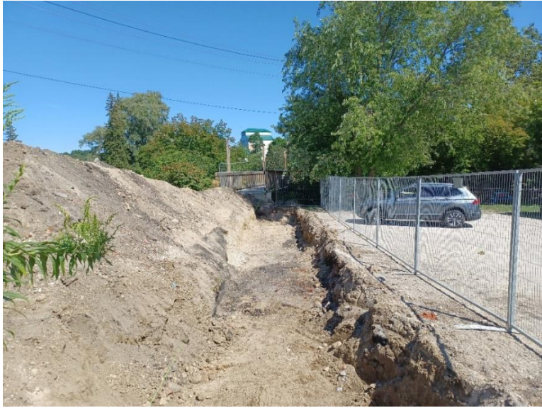
Area is prepared for construction of footings to install a new cement edge, steps and flower boxes.
