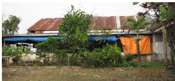
Kitchen Facility ( from outside)
