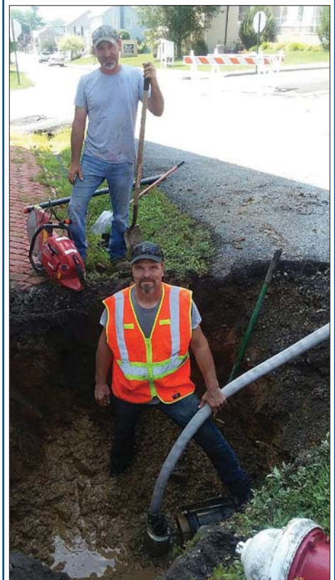
Borough employees Matt Stringer (bottom) and Randy Stoner dig their jobs—literally!
