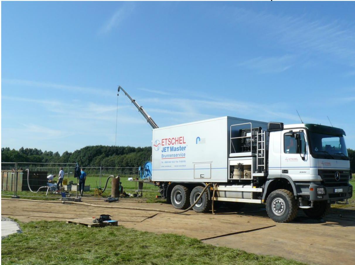
Well development with the JET Master®
