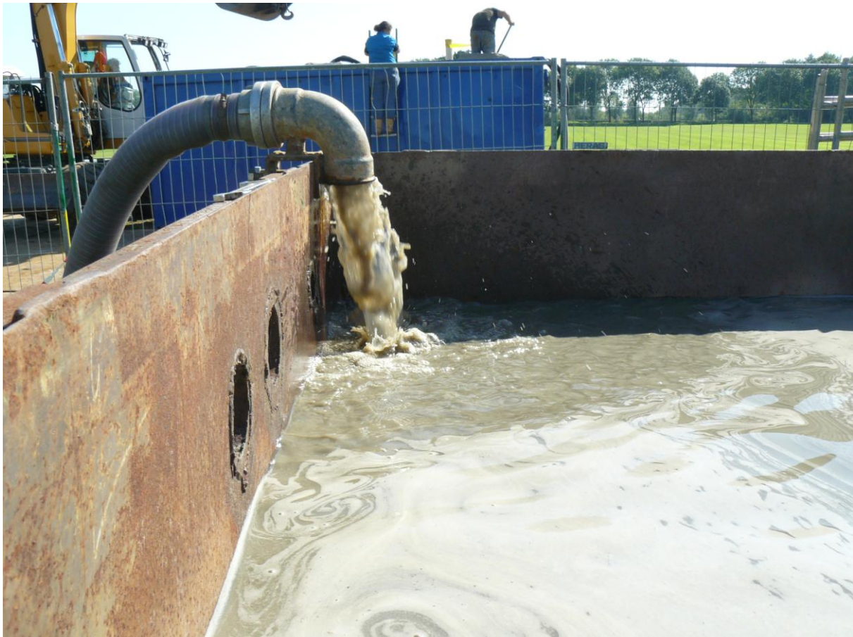
Extraction of Bentonite while developing a well with the JET Master®
