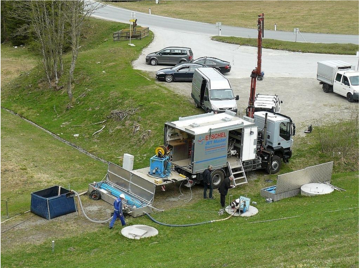
- State of the art JET Master® rehab site
