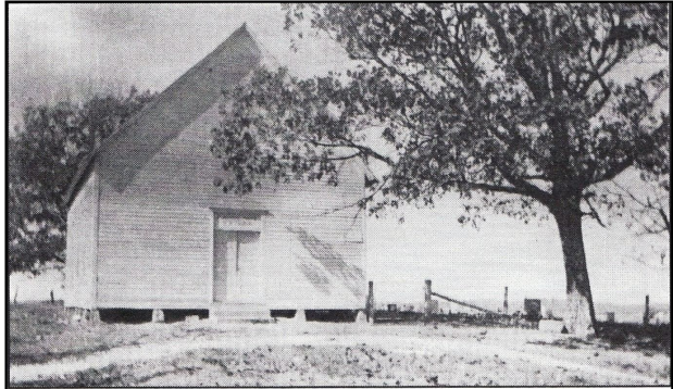
PLEASANT RIDGE CHURCH - NEAR MIFFLIN, INDIANA BUILT IN 1906 and TORN DOWN IN 1954. Picture taken by Roy Laswell in October, 1939
