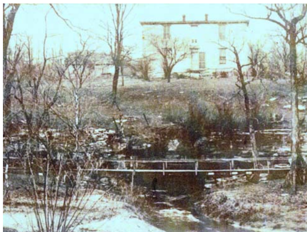
Swinging Bridge over Whiskey Run in Marengo before 1900s.
