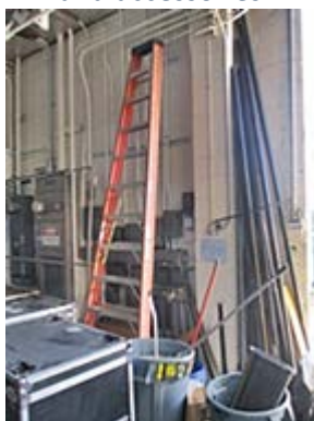
Ladder and pipes
