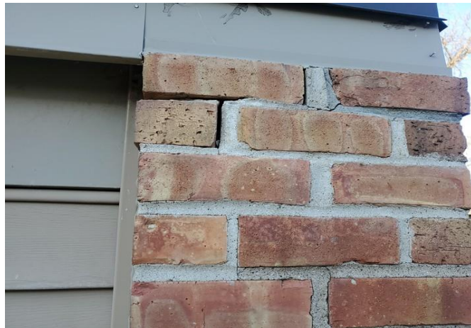
Repairs completed at edge of masonry
