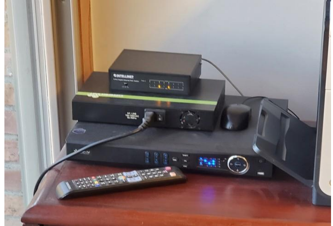
DVR and monitoring system
