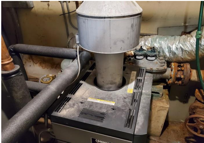
Boiler vent hood
