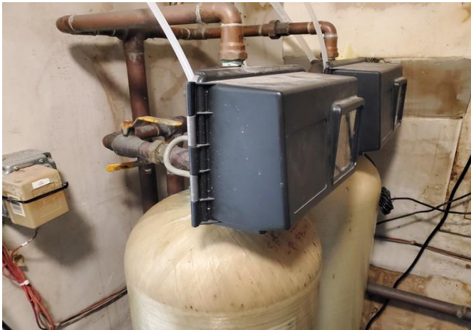
Hardware on softener
