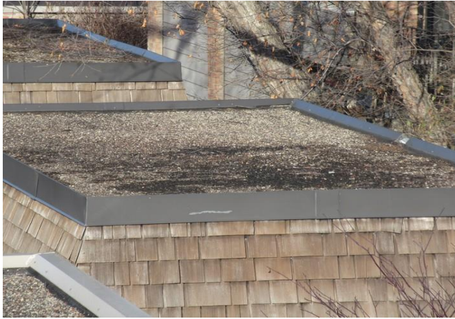
View of older ballasted roof
