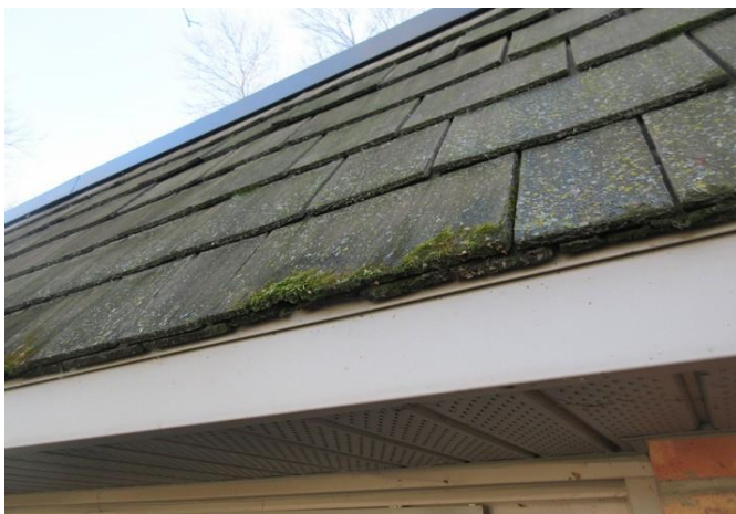
Growths on edge of roof
