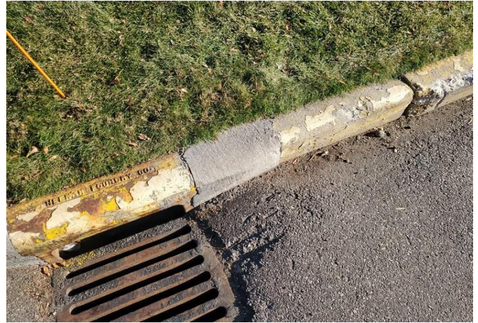
Repair at catch basin
