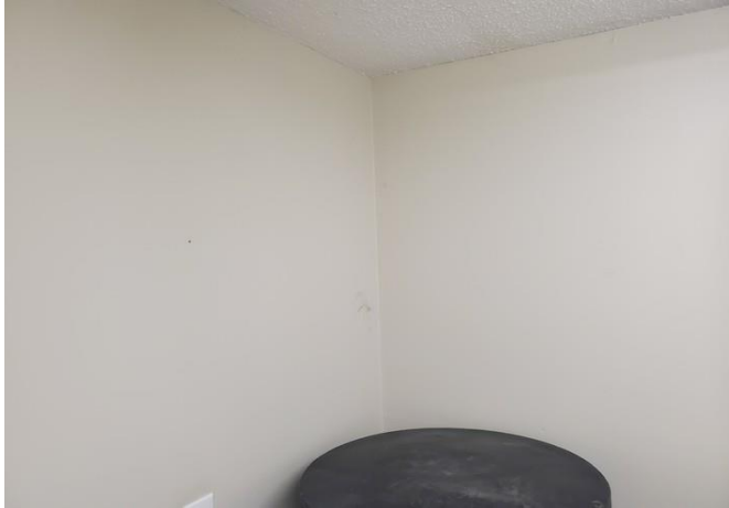
Painted walls and ceiling in common laundry
