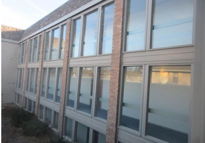
Common windows at Gallery building
