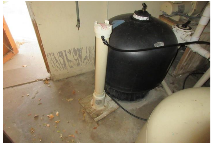
Chlorinating system and filter
