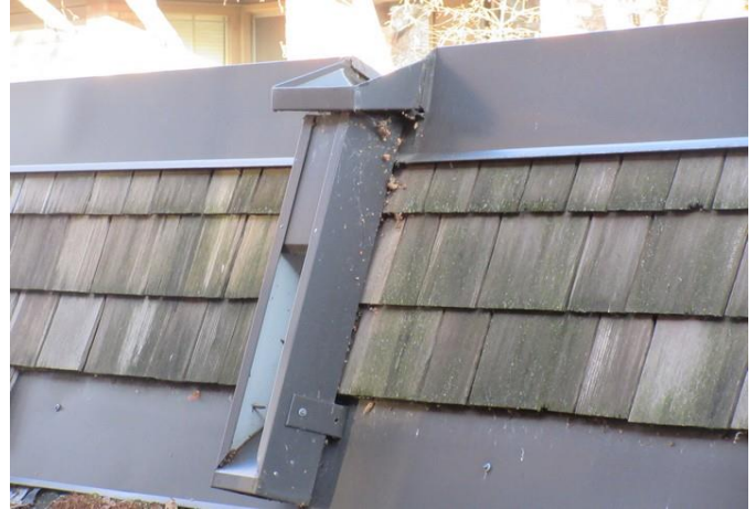
View of scupper
