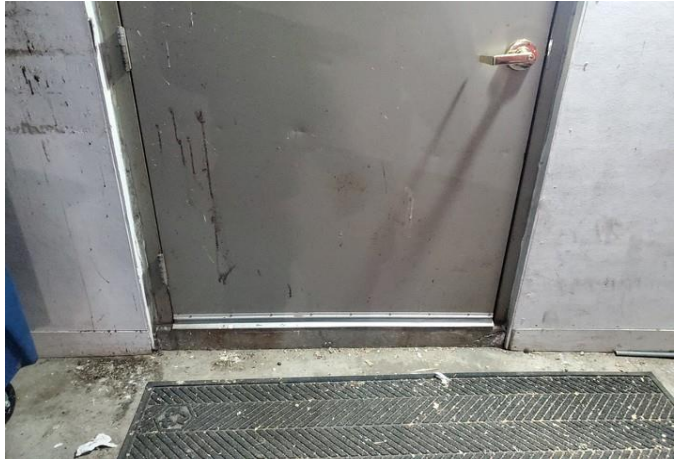
Dented and rusting door surface
