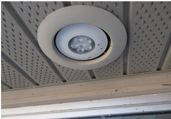
Can light at entry
