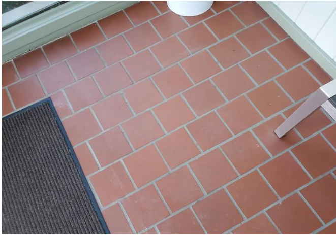
Typical tile at front entry
