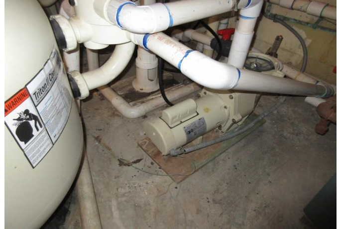
Pool pump in mechanical room
