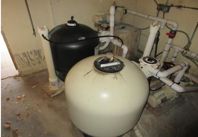
View of filters
