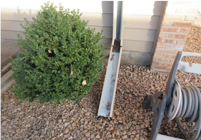
Downspout at grade
