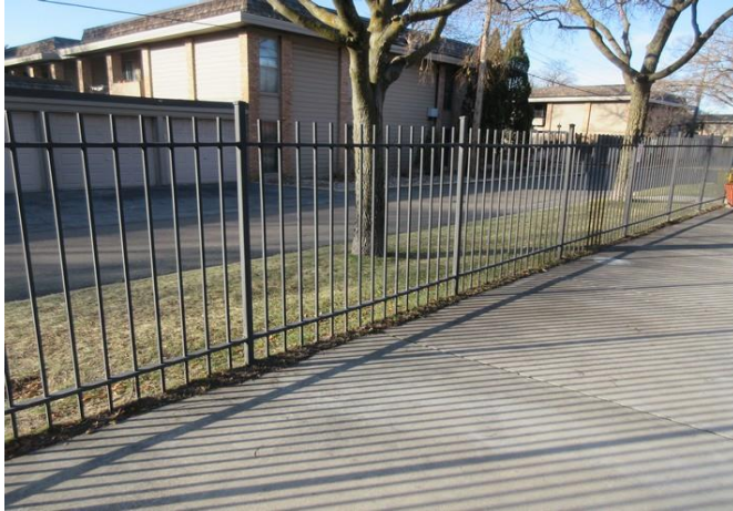
View of steel fence
