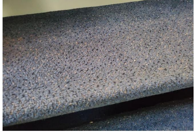
Typical condition of carpet surface
