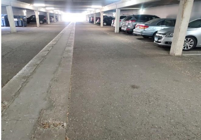
Paved garage floor
