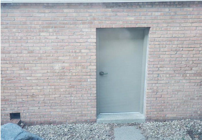
Exterior view of door to Galleries courtyard
