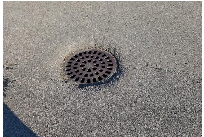
Settlement visible at catch basin
