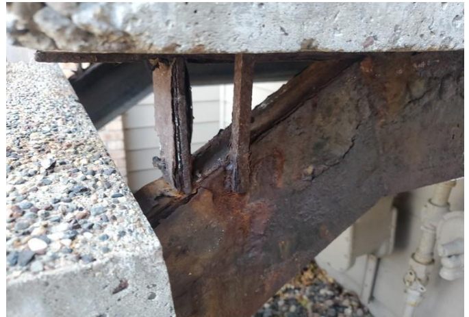
Typical condition of support steel
