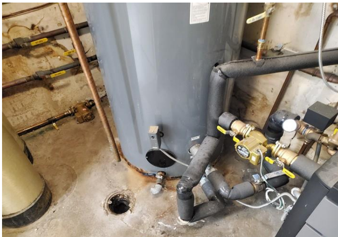
View of water heater
