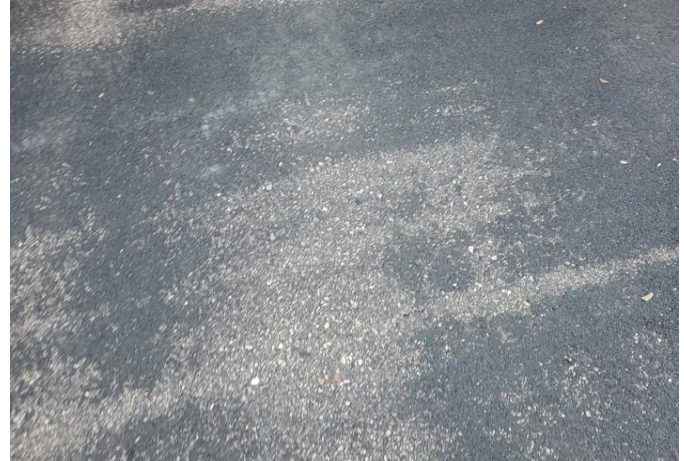
Worn seal coat
