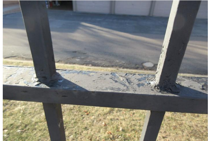
Deterioration on paint
