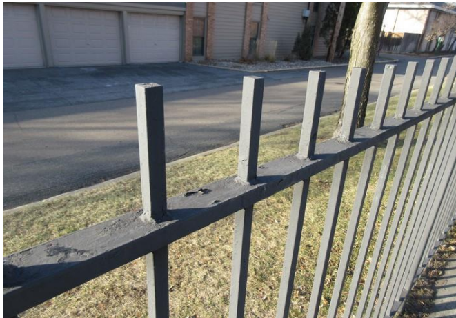
Typical condition of fence surfaces
