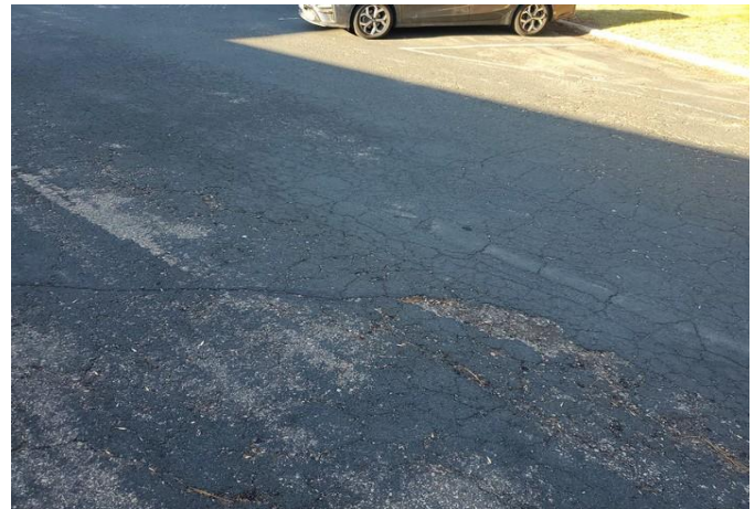
Cracks in pavement
