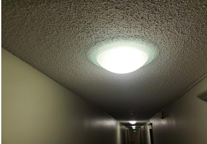
Typical hallway fixture
