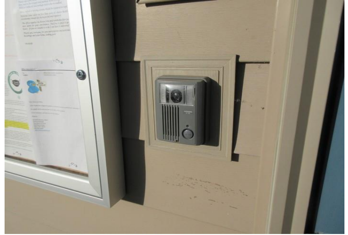
Intercom at entry to clubhouse
