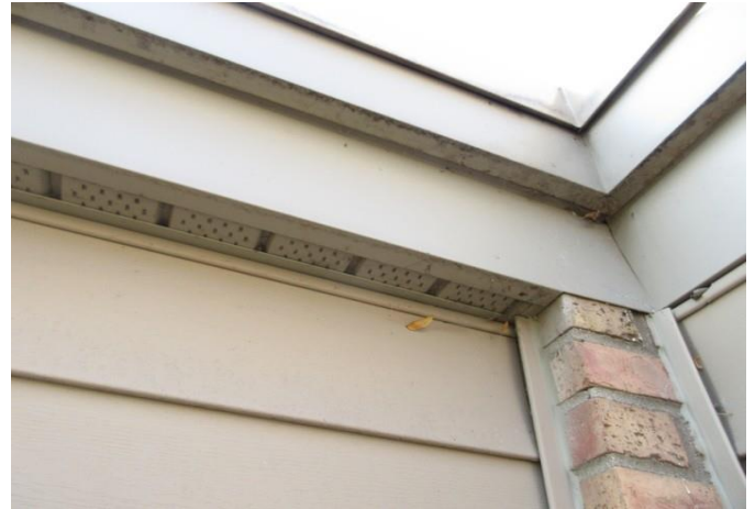
Soffits along rear of garage
