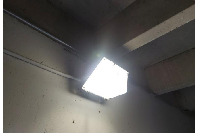
Typical wall fixture
