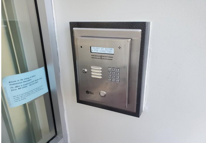
Typical intercom panel
