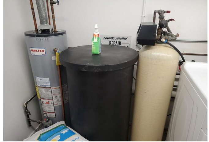
Water softener in laundry
