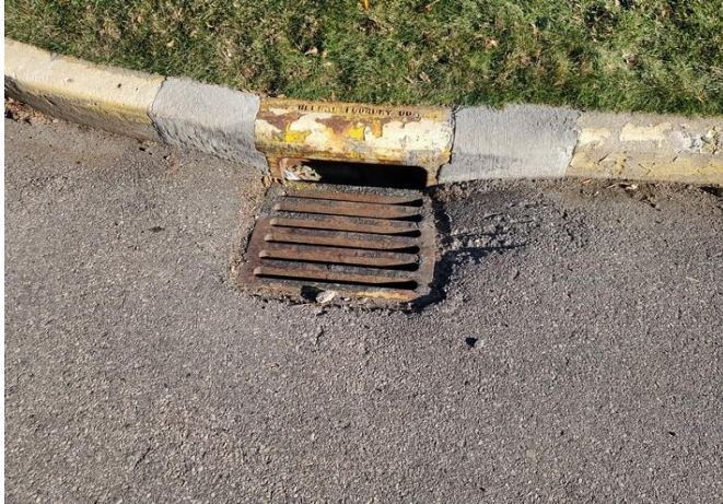
Catch basin that has been repaired at curb
