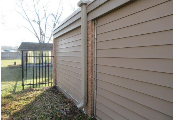
Scupper and downspout at garage
