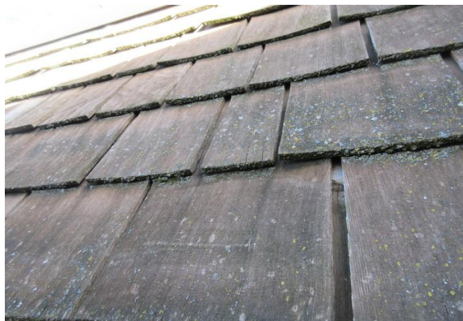
Surface of roof, with lichens growing (typical in shaded area)
