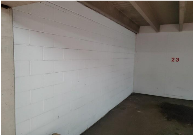
Painted concrete block
