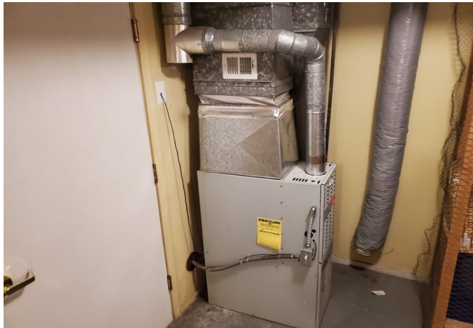
Furnace in common storage room
