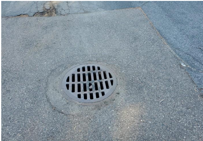
Catch basin in patched pavement
