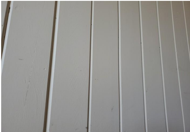
Painted wood in stairwell
