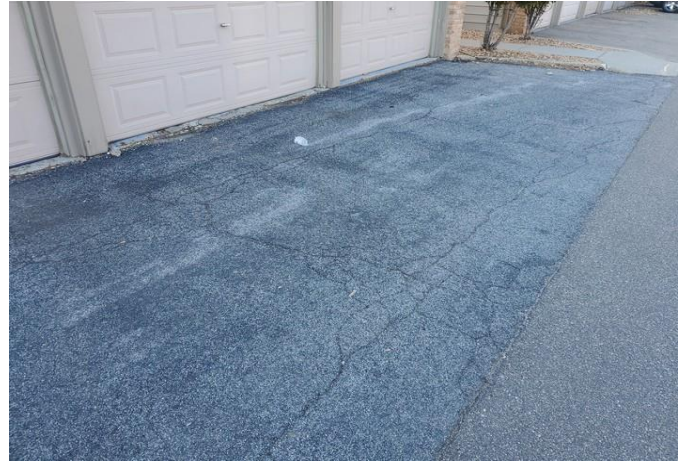
Cracked driveway pavement
