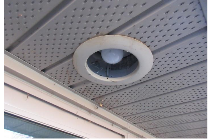
Exterior can fixture
