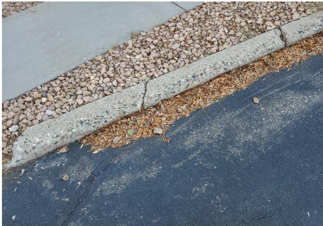
Cracks in curb
