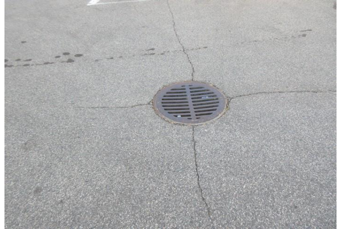
Catch basin in parking area
