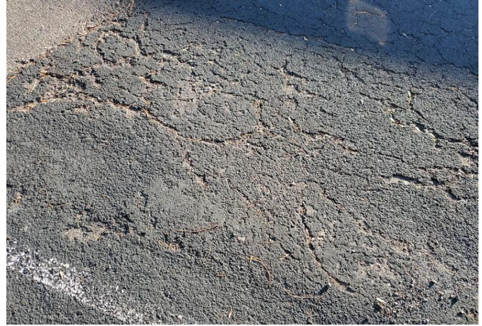
Deteriorating seal coat
