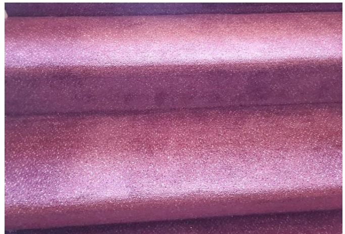
Discolored carpet due to foot traffic
