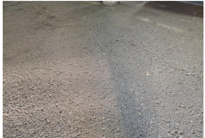
Asphalt surface in garage
