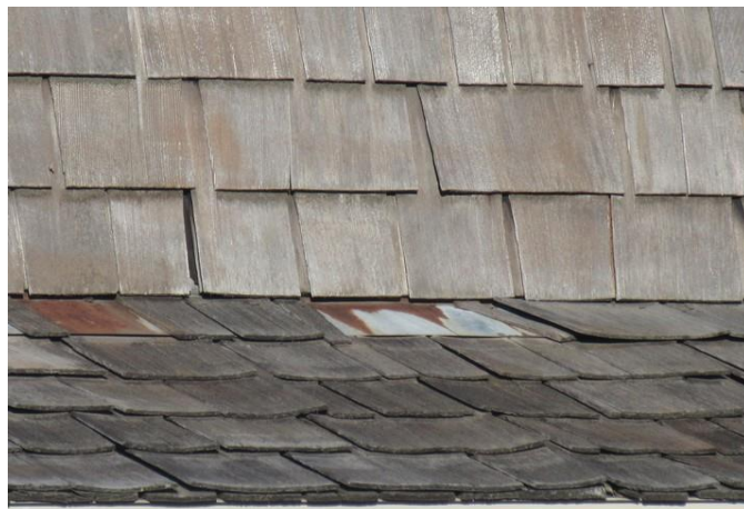
Missing shakes visible
