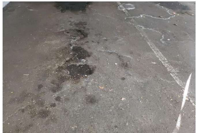
Stained and deteriorated surface
