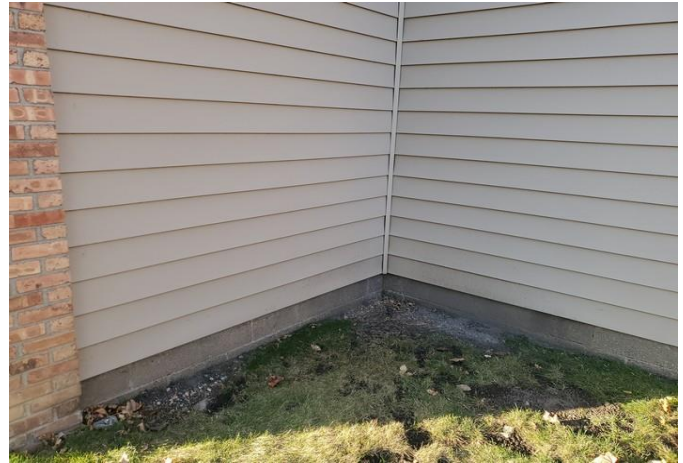
Vinyl siding at building corner
