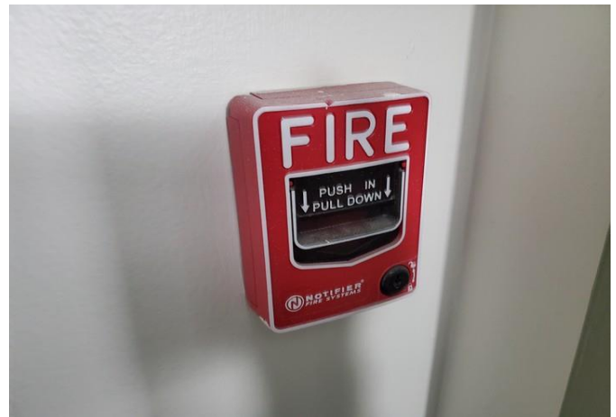
Pull station in common hallway
