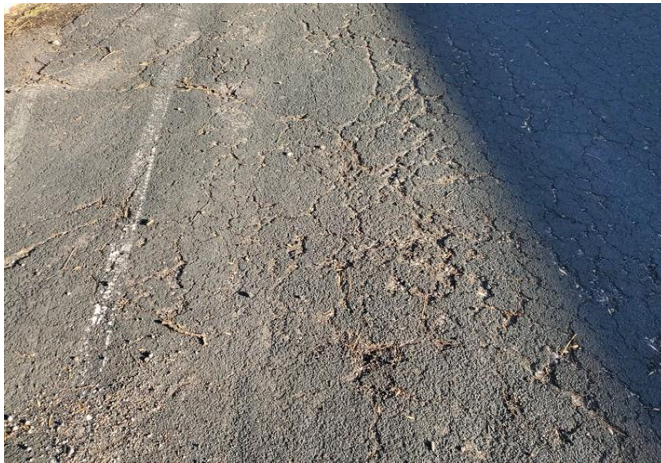
Cracking pavement
