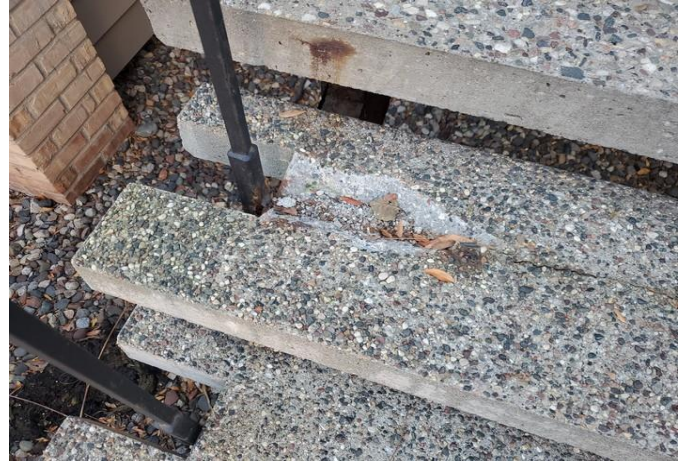
Deterioration of tread
