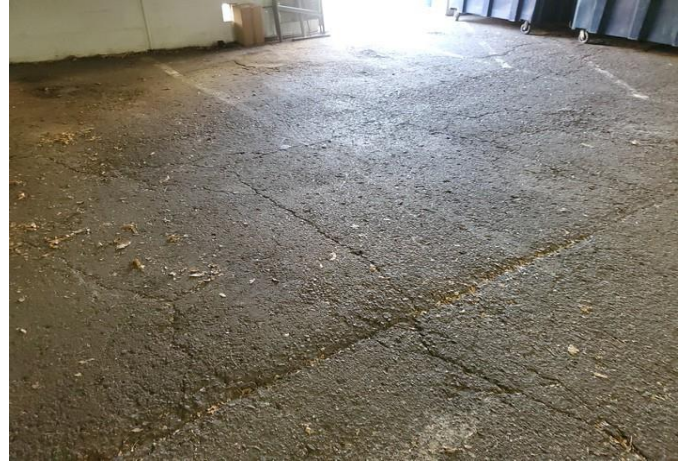
Cracks in garage floor
