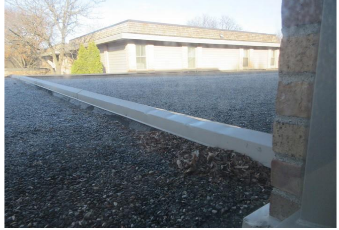
Coping and ballasted roof over garage
