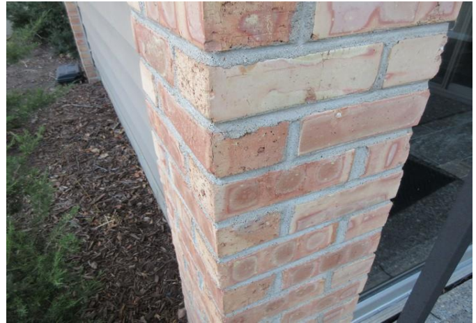
Repaired mortar at column
