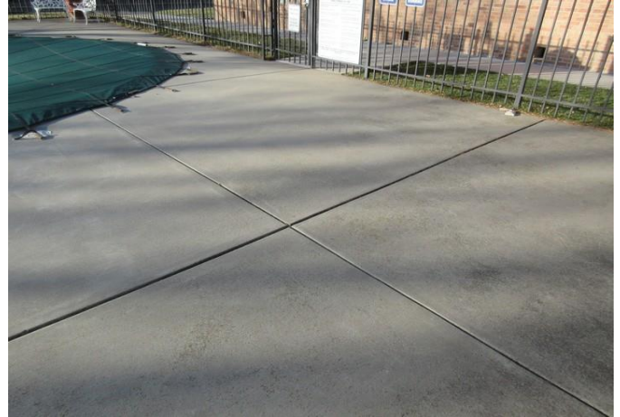
View of deck section in good condition
