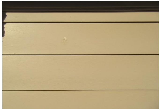
Vinyl panel siding in good condition
