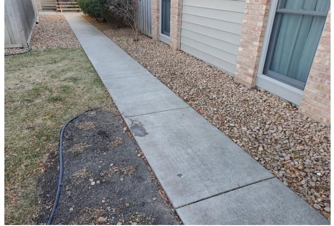
Newer concrete walk
