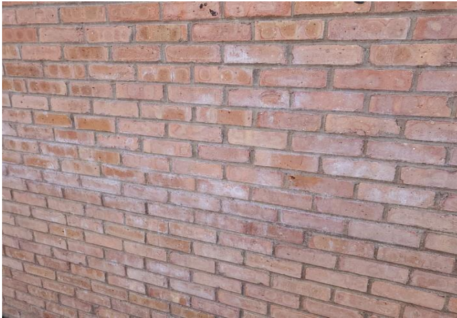
Efflorescence on brick
