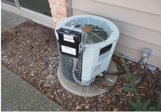
Condensing unit at clubhouse
