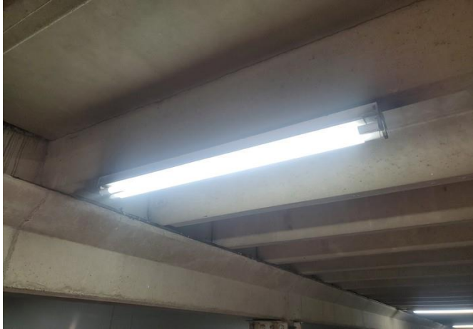
Fluorescent light fixture
