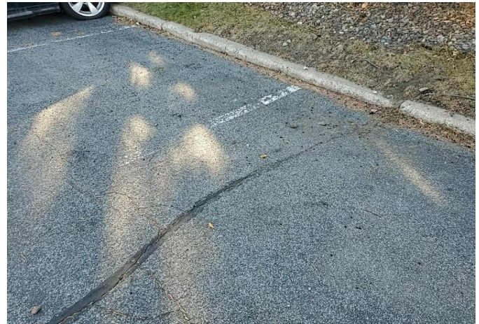
Crack in pavement near parking
