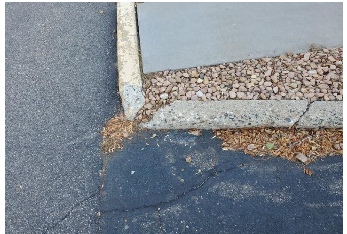
Typical condition of curb
