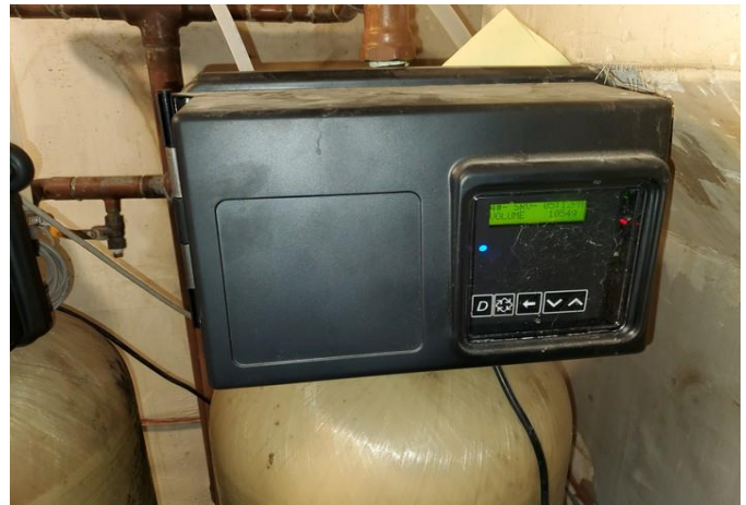
Water softener panel
