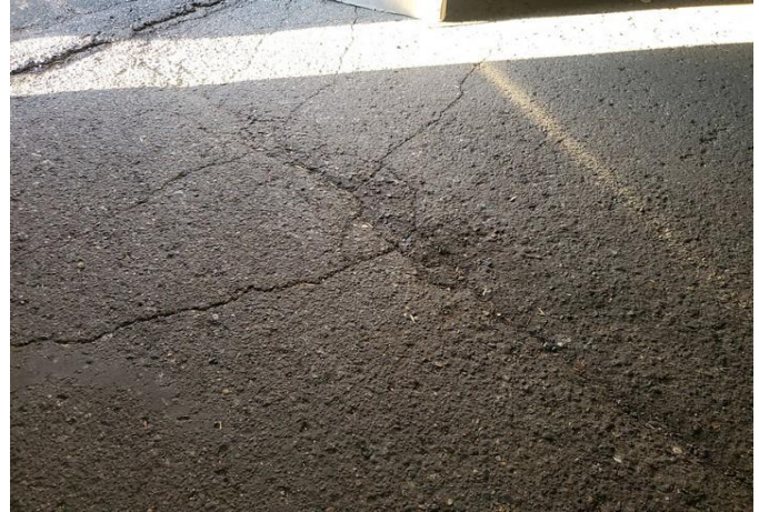
Cracks in garage floor
