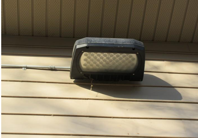
Area light at side of building
