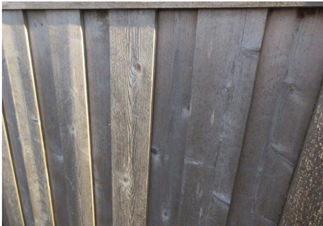
View of fence panel
