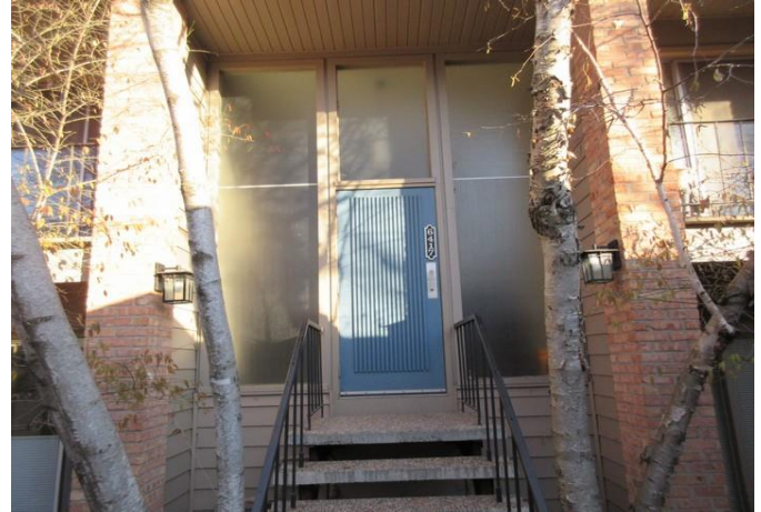
Cluster entry door and surrounding glazing
