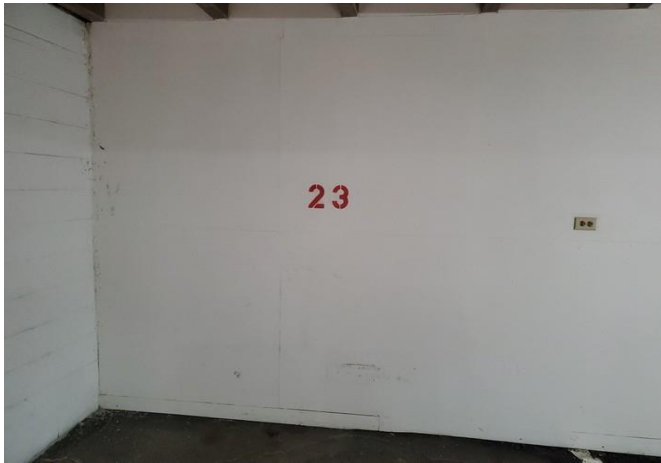
Typical wall surface
