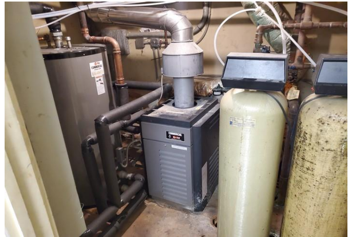
View of boiler in mechanical room
