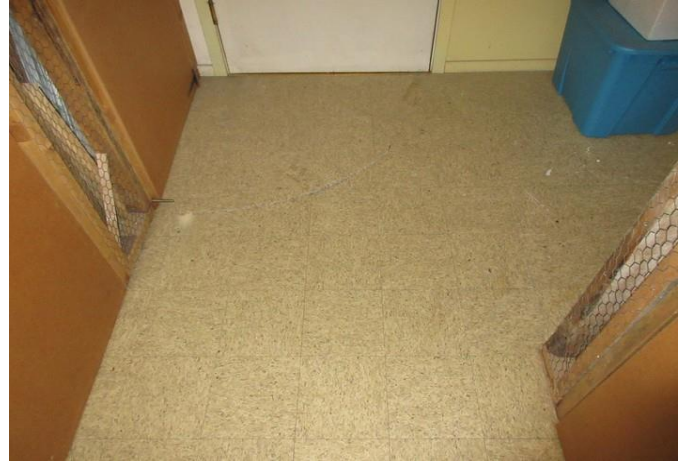
Storage area flooring
