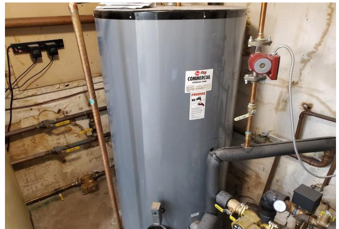
Water heater in Galleries building
