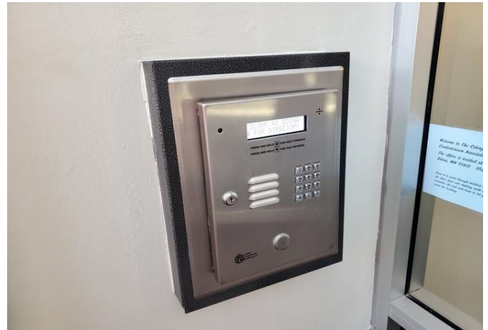
Intercom at galleries entry
