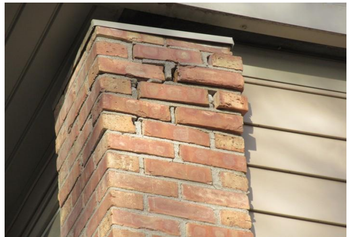
Shifted bricks and deteriorating mortar
