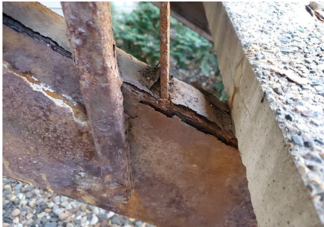
Rusted and flaking steel support
