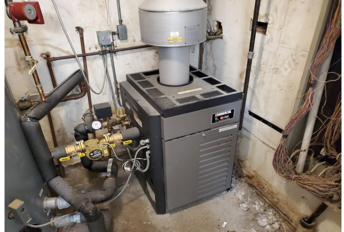
Boiler located in behind laundry room
