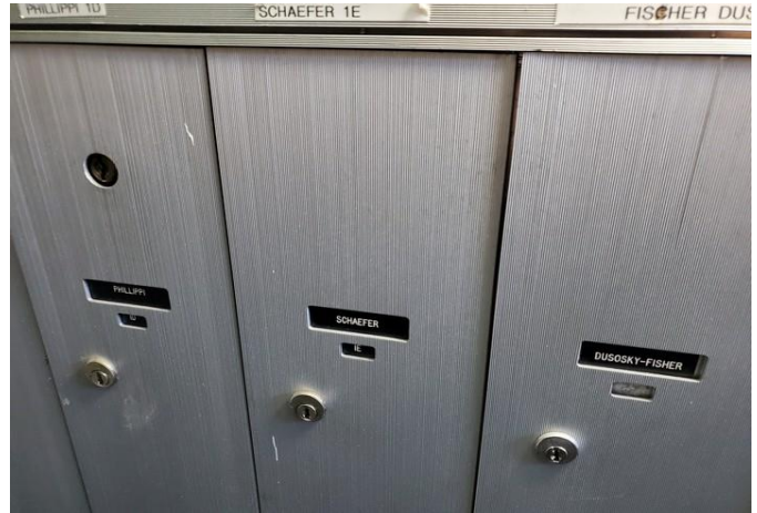
Mailboxes are in fair to good condition
