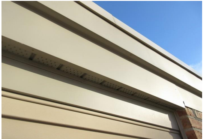
Typical fascia condition
