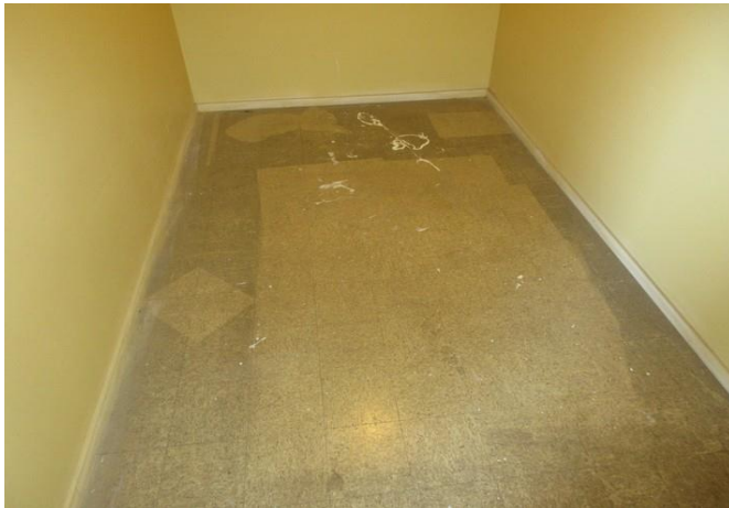
Discolored vinyl floor in storage
