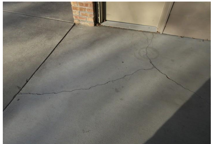
Cracked deck panels at poolhouse door
