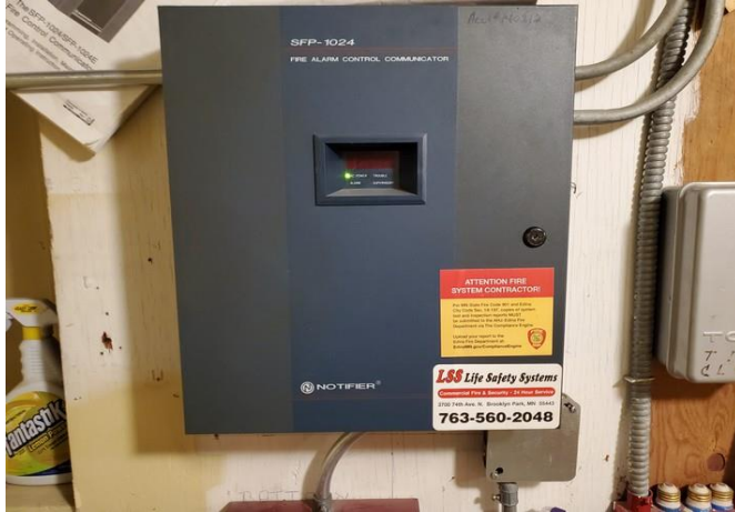
Typical fire panel in storage room
