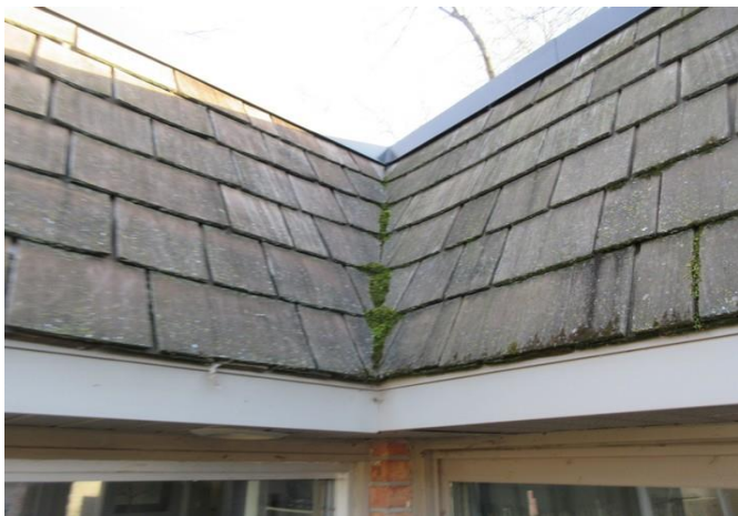
Moss growing in shake roof corner
