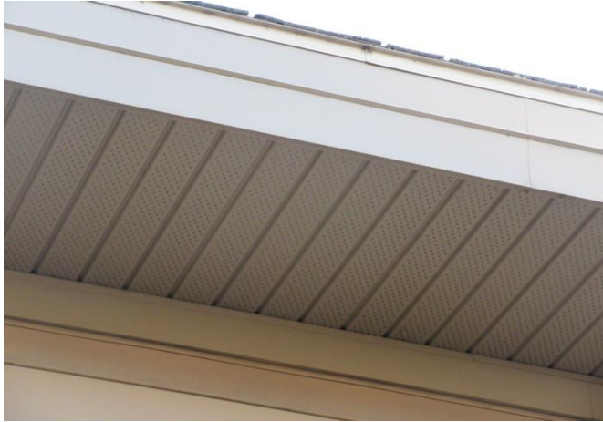
Soffit at Galleries overhang
