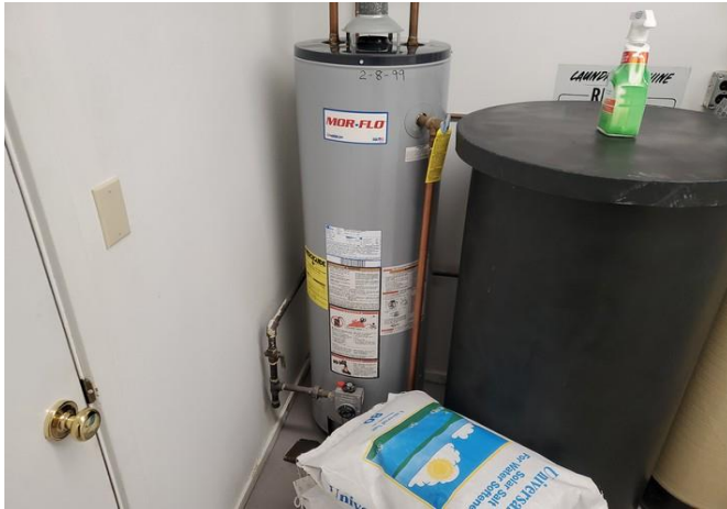
Laundry room water heater
