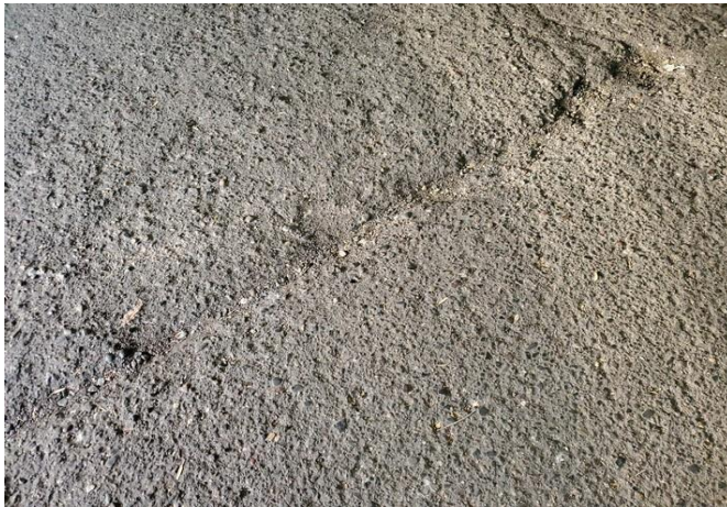
View of surface condition
