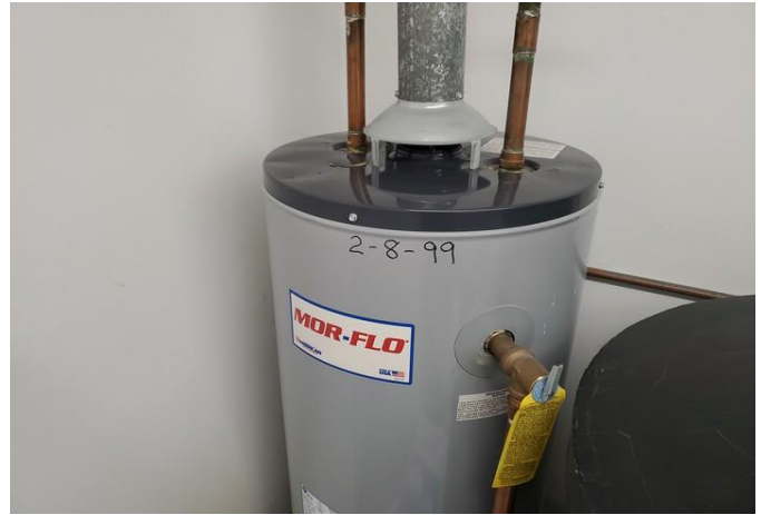
Laundry room heater with date installed shown
