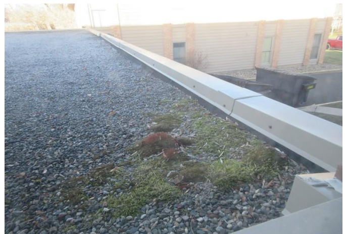
Moss growth on old roof (to be replaced)
