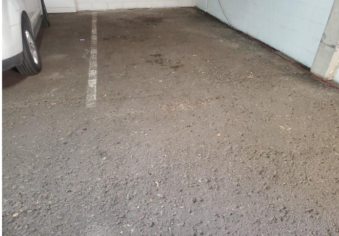
Pavement surface at parking stall
