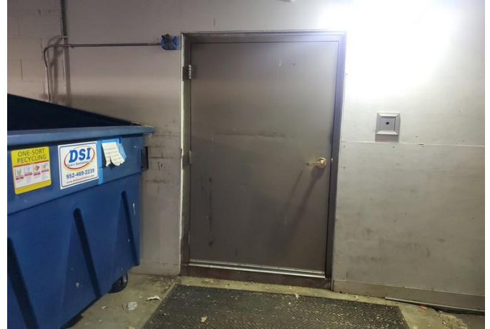
Utility door near dumpsters in garage
