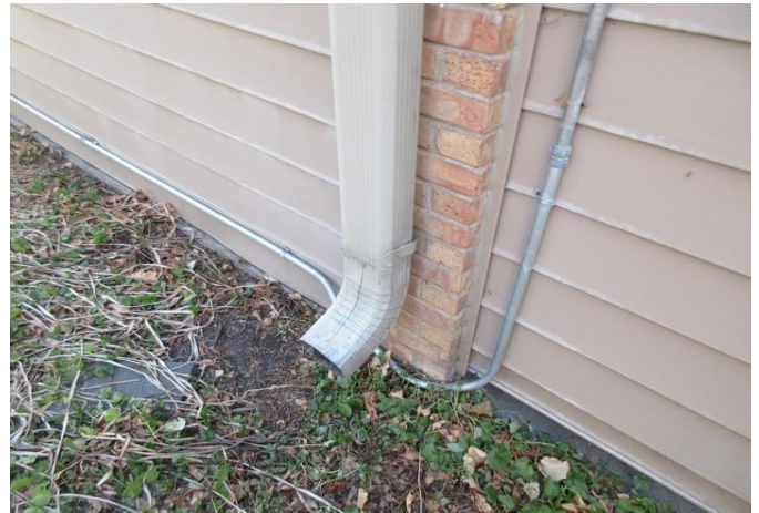
Downspout at rear of garage (note different style)
