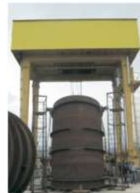
Erecting gantry crane L.c. 63/3,2t hoisting height 518m Zaramagskaya HPP (Russia)
