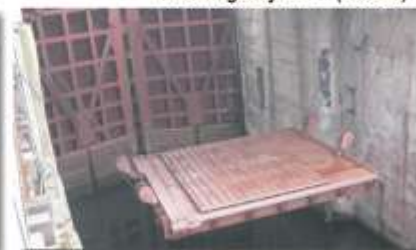
Replacement of guard gate of downstream end of Kakhovka lock
