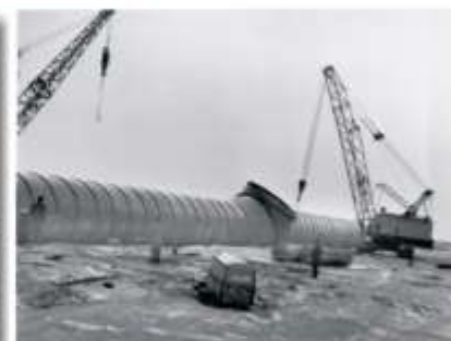
Installation of penstock of water intake structure of Zaporozhye SRPP (Ukraine)
