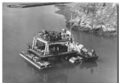
Floating station for lifting the float-type gate of Dangarian irrigation tunnel (Tajikistan)
