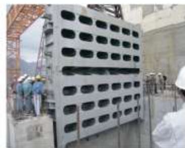
Installation of gate into the slots
