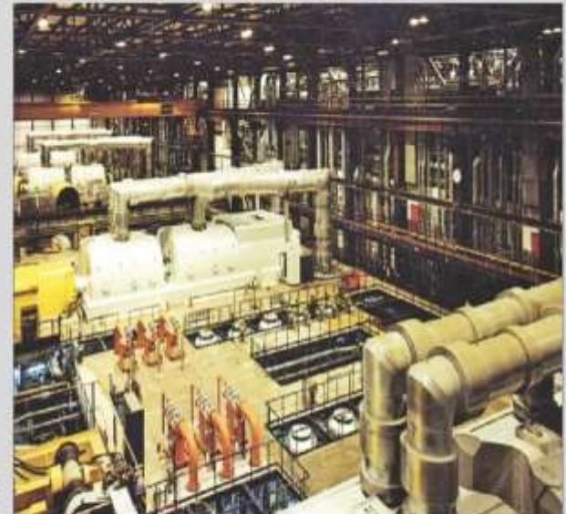
Eight turbines K-220-44 are installed at "Paks" NPP, Hungary
