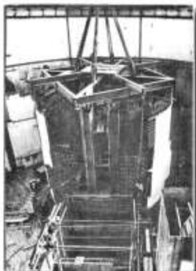
Erection of nuclear reactor vessel
