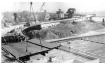
Large-size assembly of sections of highway bridge of Dneprovskaya HPP (Ukraine)
