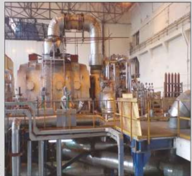
Steam turbine K-160-130 at "Puroshen" TPP, Romania
