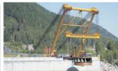
Reloading by A-frame L.c. 170t of new rotor wheels for plant units of Sayan-Shushenskaya HPP
