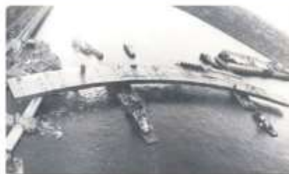
Large-size assembly of sections of highway bridge of Dneprovskaya HPP (Ukraine)
