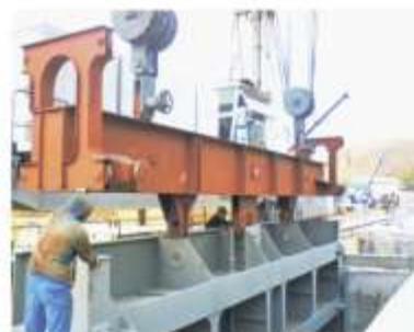
Engagement of gate by means of lifting beam
