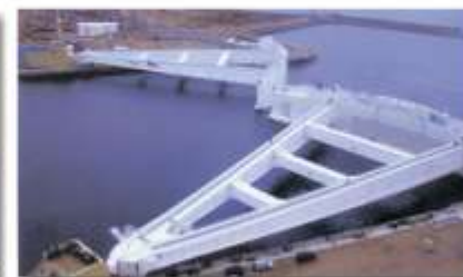
Installation of support frames of flood-gates of protective structures from overflow water of St. Petersburg city
