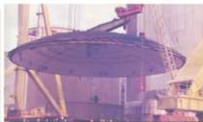
Large-size assembly of protective shell and dome of nuclear power plants
