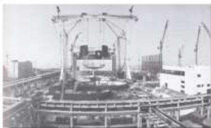
Large-size assembly of protective shell and dome of nuclear power plants
