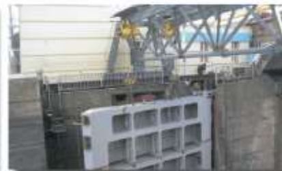
Installation of service gate leaf of the lock by means of special mounting mechanism
