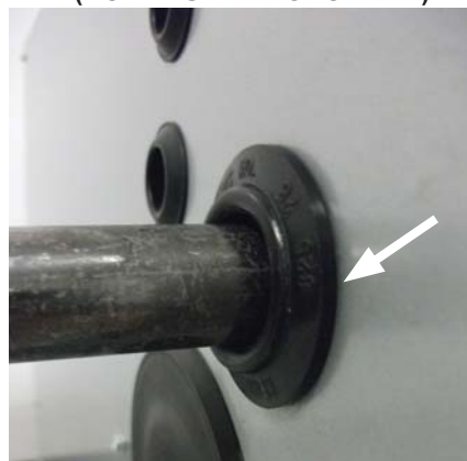
FIGURE 27 - FURNACE GAS PIPE CONNECTIONS (NOTE RUBBER GROMMET)
