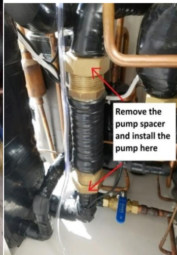
Removing the shipping spacer
