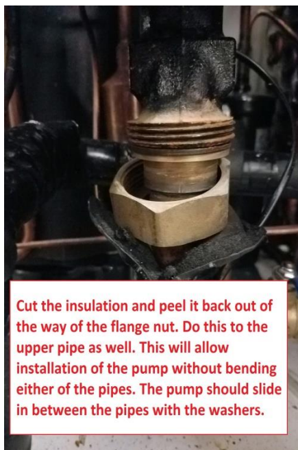
Peel back the insulation
