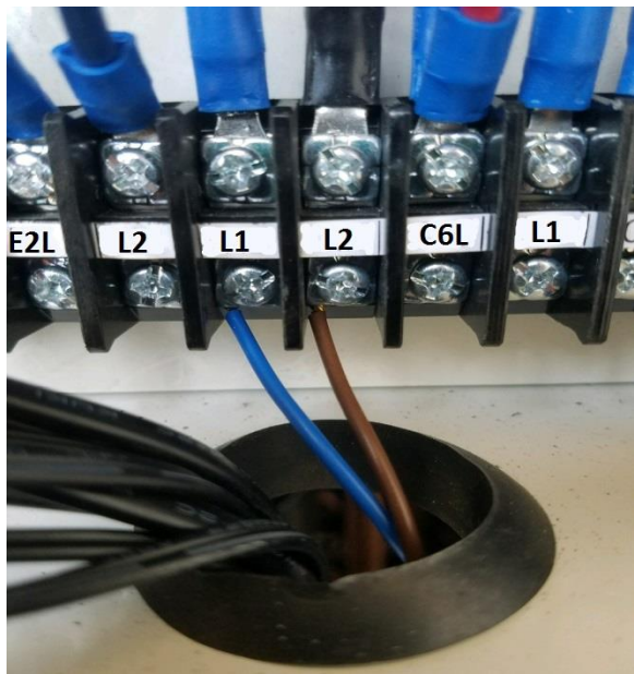
Pump power wires.
