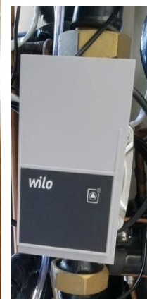
Removing the shipping spacer
