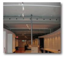
The building owner decided to go with Hi-Velocity equipment so that the ceiling height could be maintained and no structural changes would be needed to the building. Energy Saving Products Ltd. Hi-Velocity System was the ideal choice, the round plenum runs on the ceilings with drilled outlets were easily installed. Using drilled outlets in the plenum was cost effective, and allowed for a fast setup time.
