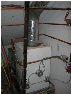
A total of seven tons of cooling is conditioning this building. In this application two Hi-Velocity units installed in the vertical position (up-flow) were used, a HV-70 and a HV-100. They were easily placed in out of the way places, as the Hi-velocity System does not need to be centrally located.
