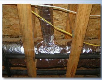
The two inch ductwork results in less custom sheet metal work, minimizing waste and provides the flexibility for complex architectural designs. The high moisture removal of the Hi-Velocity Systems will remove up to 30 percent more humidity from the air, providing greater comfort while eliminating the cold clammy feeling that can exist with conventional systems.
