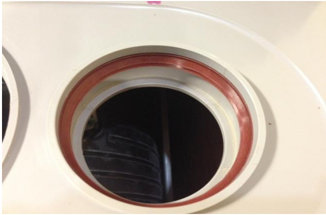
Figure 2 Air intake of a two pipe system after white cap is removed. It is on the right side of boiler
