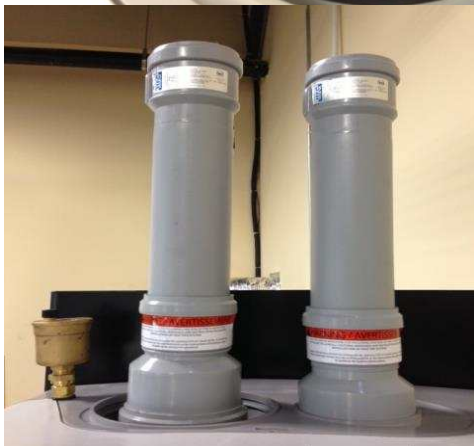
Figure 4 After O-rings are installed, connect polypropylene venting as pictured. Use 3" or if short vent length, reduce to 2" as seen in picture. See vent chart below for max vent lengths.
