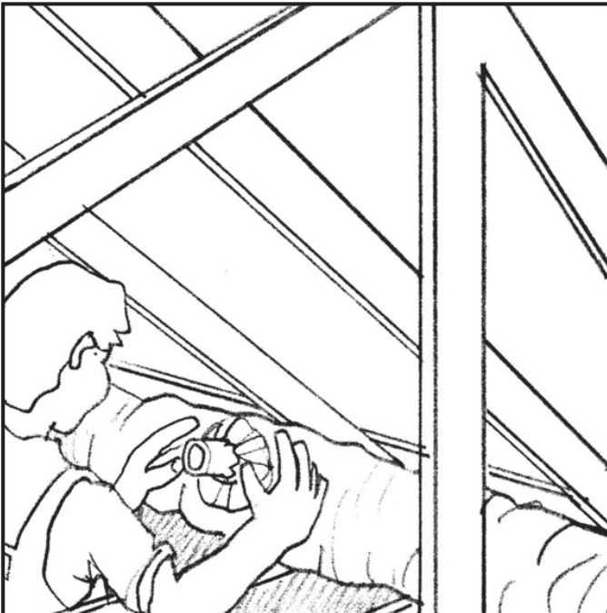
Fig. DUC-11 - BTO with insulation sleeve
