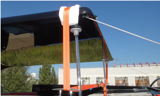
Pic. 28: Abandoned roof supported by supports, fastened by a transport belt
