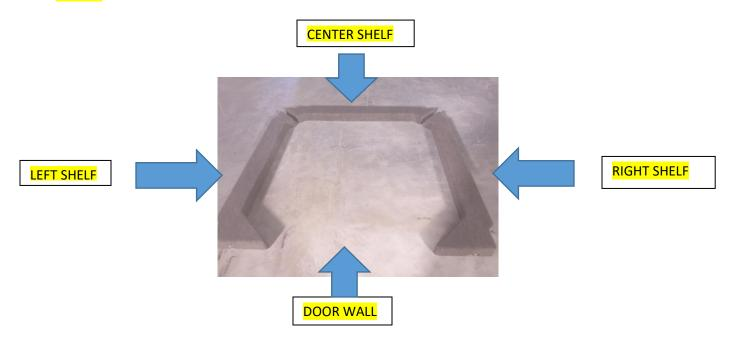
STEP 2 – INSTALL ONE OF THE REMAING SHELVES ON THE SIDE [BUTT THE MATCHING END OF THE SHELF UP TOO THE END OF THE SHELF ALREADY INSTALLED IN THE CENTER WALL] THESE SHELVES FIT VERY TIGHT AND WILL TAKE A LITTLE EFFORT TO ALINE UP WITH THE BOLTS HOLES IN THE WALL [IF NEEDED TAKE A SMALL SCREWDRIVER AND STICK IT THRU THE OUTSIDE WALL BOLT HOLE AND THE CLIP NUT ON THE SHELF TO HELP LINE IT UP.] REPETE STEP 2 FOR THE REMAINING SHELF.
