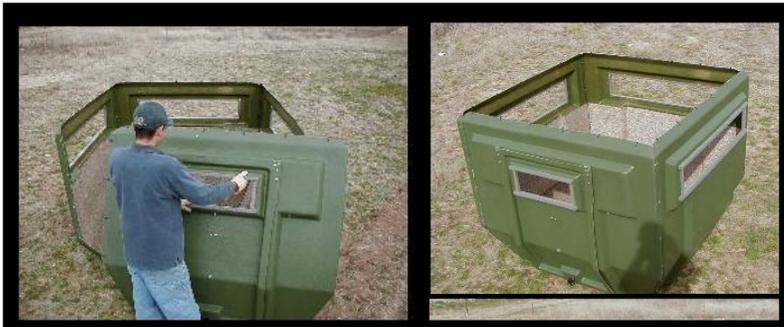
7. Move the carpeted floor section into the partially erected blind and lay it down so that the holes in the floor are over the holes in the foot sections of the wall panels. **NOTE- The floor must go on top of the wall panel feet, not underneath.** This is very important from a safety standpoint.
