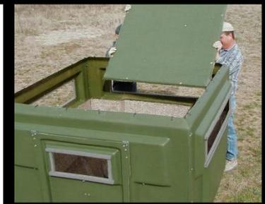
8. Place the roof on top of the four panels. Insert the bolt / metal washer / neoprene washers through the roof panel and into the clip nuts on the top edge of the wall panels. Note –the bolt kit contains several longer bolts for the corner holes in the roof, these bolts at the corners should be inserted first. Once these eight bolts have been started the other roof bolts can be inserted.
