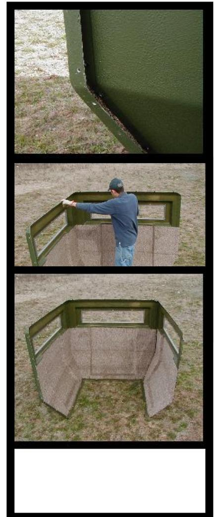
6. Then attach the door panel and secure it the same way. At this point you should have the three window wall panels and the door panel standing and loosely attached to each other.
